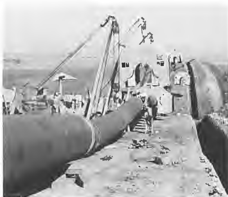
Automatic welding along the Eastern Leg near Jenner, Alberta.
