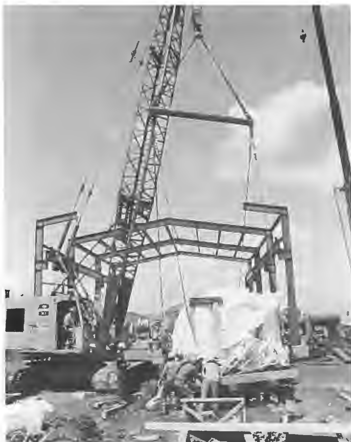
An electrically-driven compressor, the second unit for the Jenner, Alberta compressor station, is moved into place.
