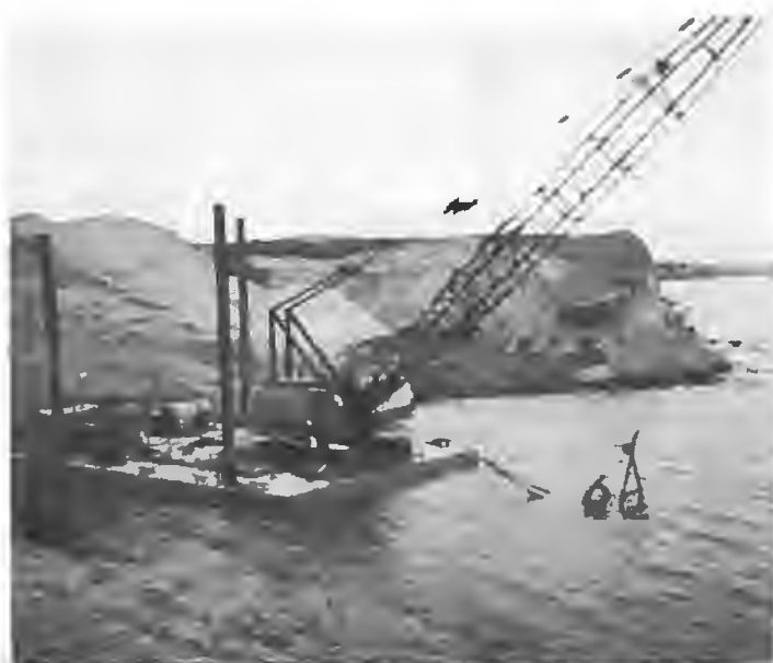
Trenching for the pipeline crossing of the 1820-m (6,000 ft.) wide Oahe Reservoir along the U.S. Eastern Leg in North Dakota, using a "clammer" mounted on a barge.
