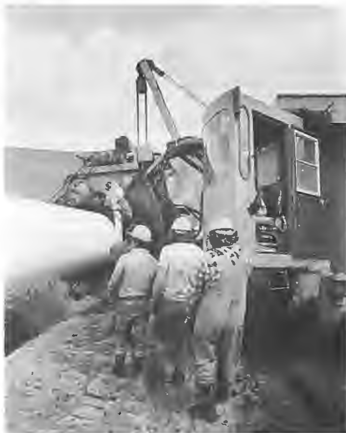
Test run near Standard, Alberta of a prototype coat and wrap machine which uses state of the art technology for hydraulic operation and electronic controls.
