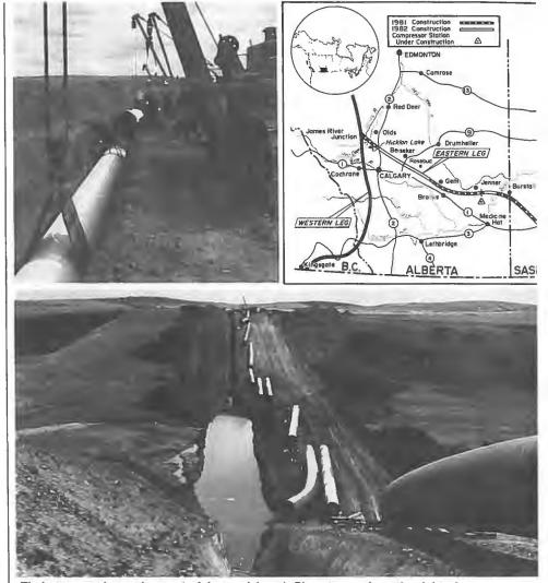
Tie-in to a road crossing east of Jenner (above). Pipe strung along the right-of-way and ditch prepared for crossing Severn Creek near Rosebud (below).
