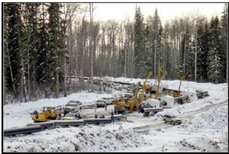
A typical gas pipeline winter construction right of way.
