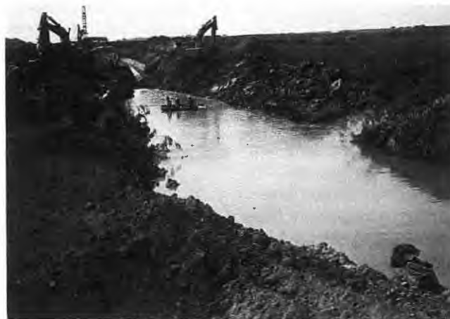
Foothills inspectors check the depth of the ditch for the pipeline crossing of Serviceberry Creek along the Eastern Leg in Alberta.
