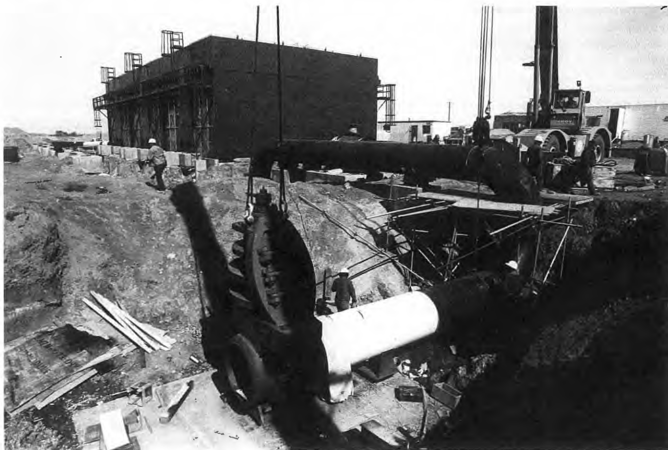
An orifice plate is lowered into the yard piping system to measure gas volumes and pressures at the compressor station under construction at Piapot, Saskatchewan.
