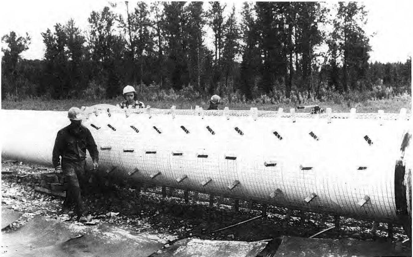
Construction crews wrap the pipe in wire mesh prior to its encasement in concrete.
