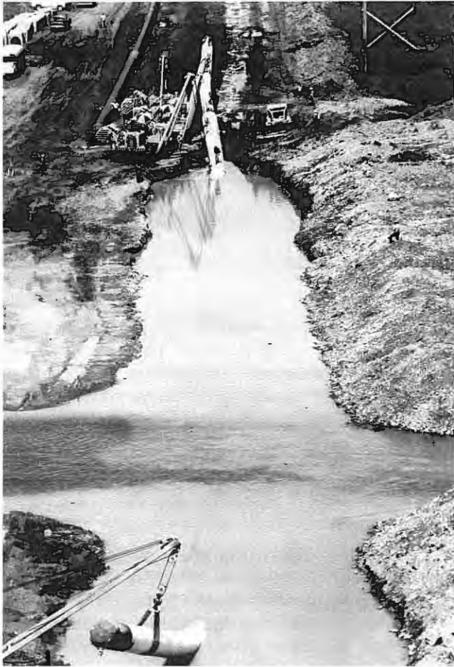
Sideboom tractors lower the pipe into the river bed during Eastern Leg construction.
