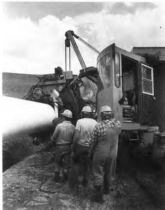
Test run near Standard, Alberta, of a prototype coat and wrap machine which uses state of the art technology for hydraulic operation and electronic controls.
