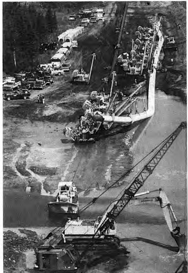
Construction crews prepare to lower the pipe into the river bed during Eastern Leg construction.
