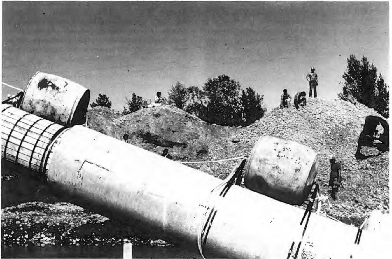
In preparation for a major river crossing, floats are attached to the pipe to maintain buoyancy while pulling the pipe across the body of water.
