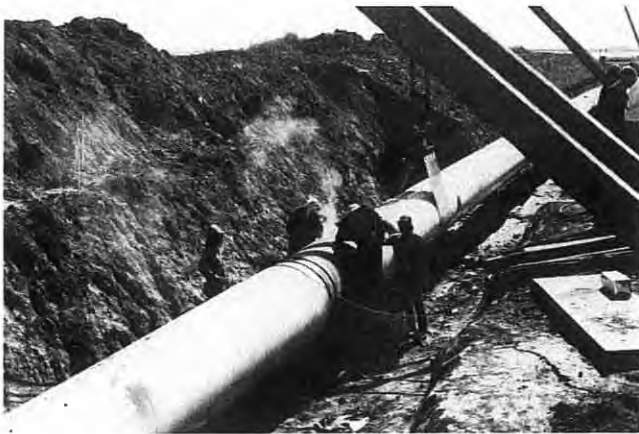
The final tie-in weld, completed on August 17, 1982, south of Beiseker, Alberta, wraps up construction of the Eastern Leg of the pipeline in Canada.
