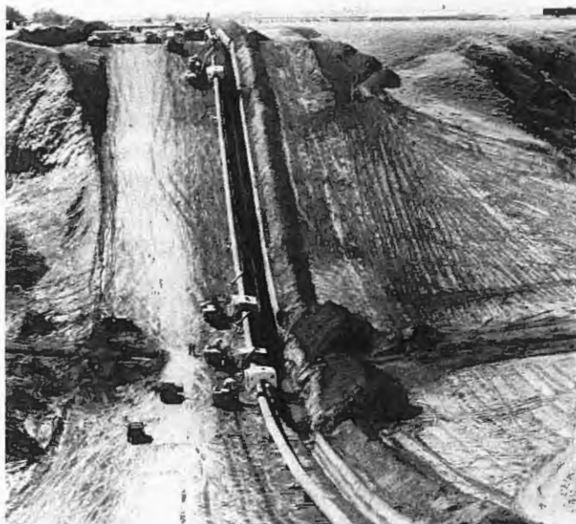
Automatic welders move down the 45-m (140 ft.) deep west bank of Irishman's Coulee in eastern Alberta.
