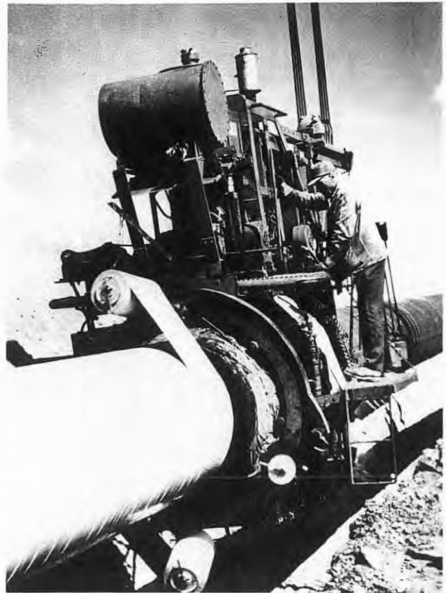
Wrapping operations at the pipeline crossing of the South Saskatchewan River in eastern Alberta.
