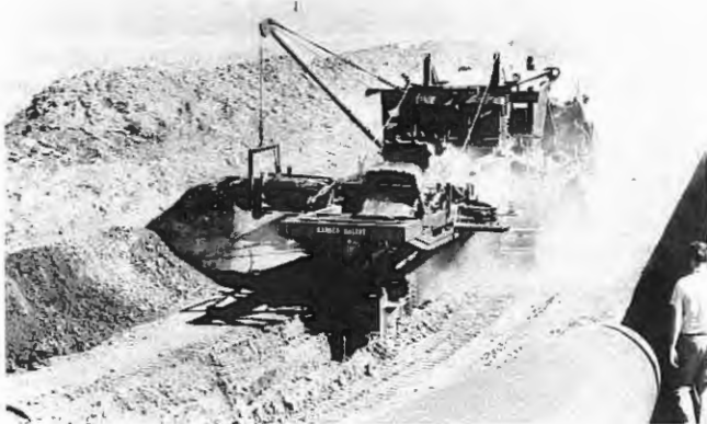
Ditching in the Great Sandhills of Saskatchewan. This ditcher is capable of digging a trench three-m (10-ft.) deep and two-m (6.5-ft.) wide to allow for a minimum of 0.8-m (three-ft.) of cover over the pipe.
