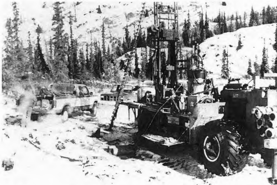
Geotechnical crew sets up drill to take core sample along the Alaska Highway near Marsh Lake in Yukon.
