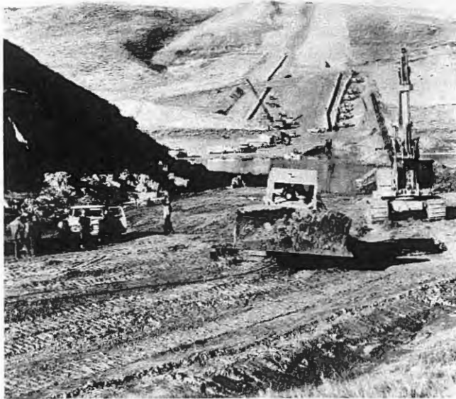
Crossing the South Saskatchewan River in eastern Alberta. As sideboom tractors lower the first section of pipe into the water, a bulldozer anchored on the opposite shore pulls the pipe with cables.
