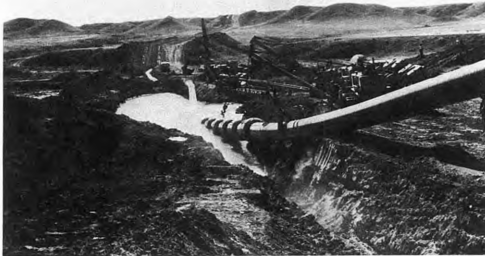
Sideboom tractors lower the pipe into the bed of the Frenchman River in southwestern Saskatchewan.
