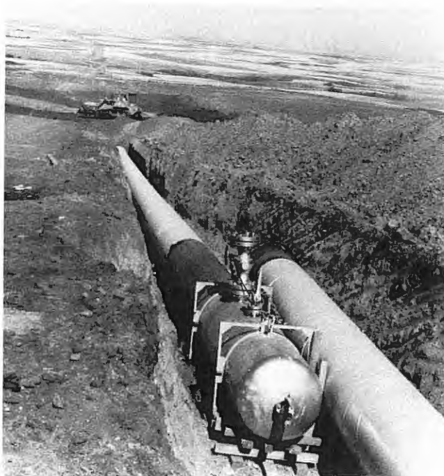
A completed pipeline section is ready for hydrostatic testing near Piapot, Saskatchewan. Heavy-walled test heads welded onto the pipe end are designed for safety as the water inside the pipe is pumped to test pressure—a minimum of 10 863 KPa (1,575 psi).
