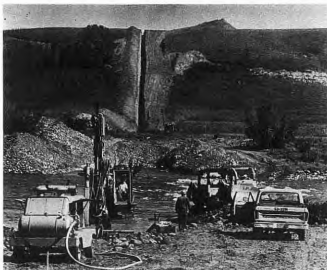
Drilling the ditch through the bed-rock of the Bow River, west of Calgary, in preparation for the installation of the pipe.
