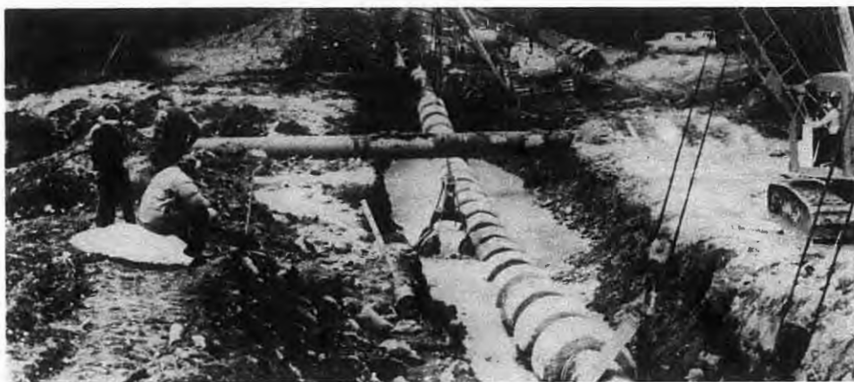
A flume is installed across the TeePee Creek in southern B.C. before the pipe is installed.
