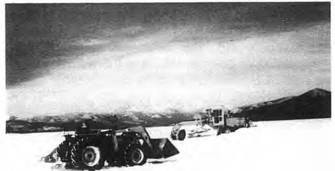
As part of the Quill Creek test program, an experiment was carried out using ice as a protective road-bed over permafrost. Shown above, a large roto-tiller attached to a farm tractor harvests ice chips from Kluane Lake for use in access road construction.
