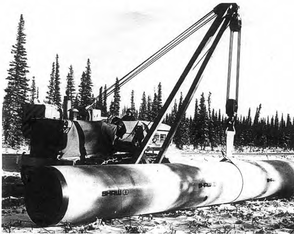
Sidearm tractor manoeuvring pipe at the Foothills' Quill Creek test project near Kluane Lake, Yukon.
