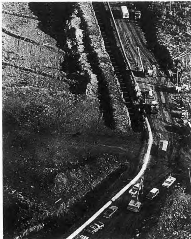
Pre-heaters warm the pipe, ahead of the wrapping and lowering-in crews in Southeastern B.C. Styrofoam supports in the ditch protect the pipe from rocks in the trench.
