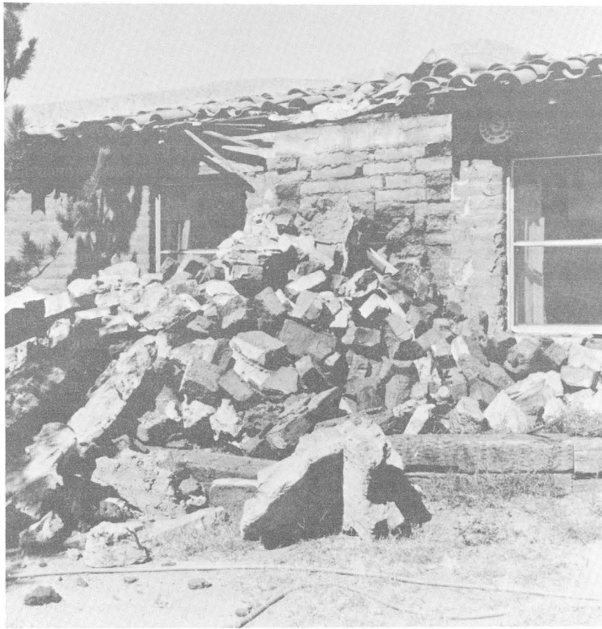
Figure 14. A fallen chimney in Whitewater Canyon, California (Borchardt and Manson, 1986).
