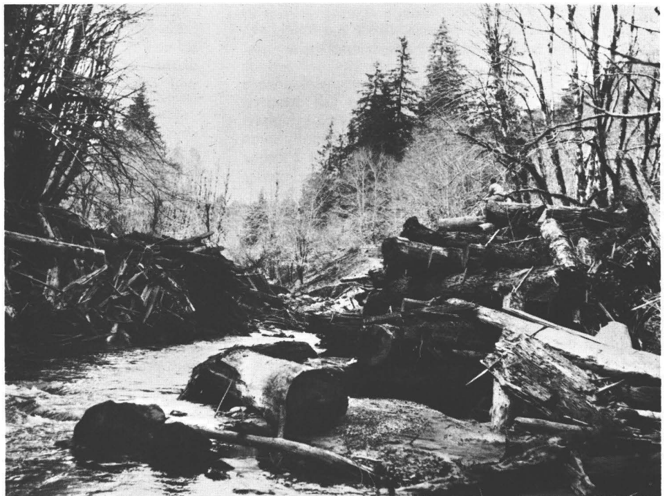
Figure 14.—Old crib dam on South Yamhill River, Oreg., after removal.
