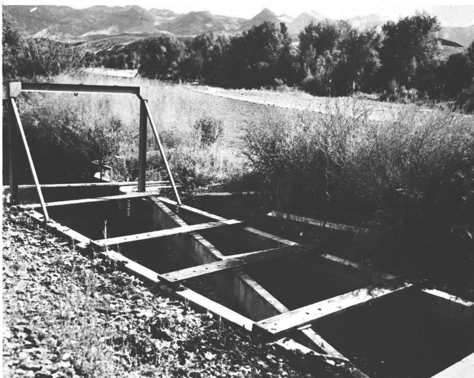
Figure 16.—Louver fish screen located in an irrigation diversion from the main Salmon River near Salmon, Idaho.
