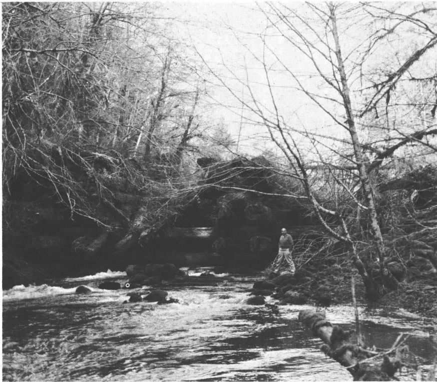
Figure 13.—Old crib dam on South Yamhill River, Oreg., before removal.
