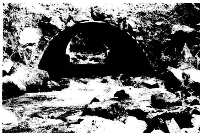
Figure 1.--Pipe arch used to allow fish passage.
