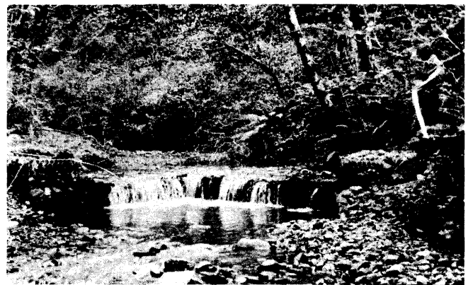
Figure 5.--Reverse V gabion.
