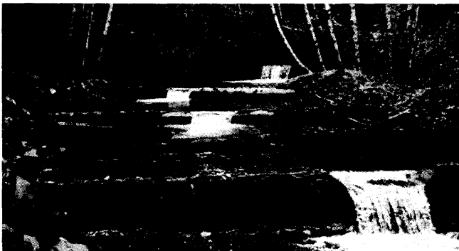
Figure 3.--Log weirs used to correct a culvert entry barrier.
