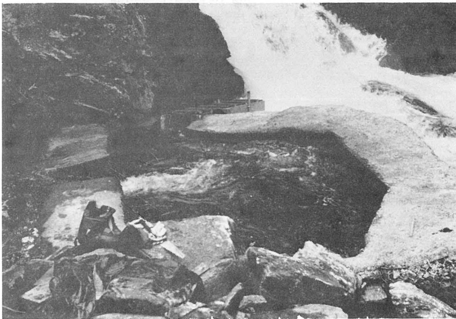
NEW ENTRANCE--A new gabion, concrete entrance pool and 10 foot steep pass section were constructed at Paul's Lake Ladder in 1976. The new pool eliminates an entrance problem that delayed passage of 26,000 sockeye the previous year.
