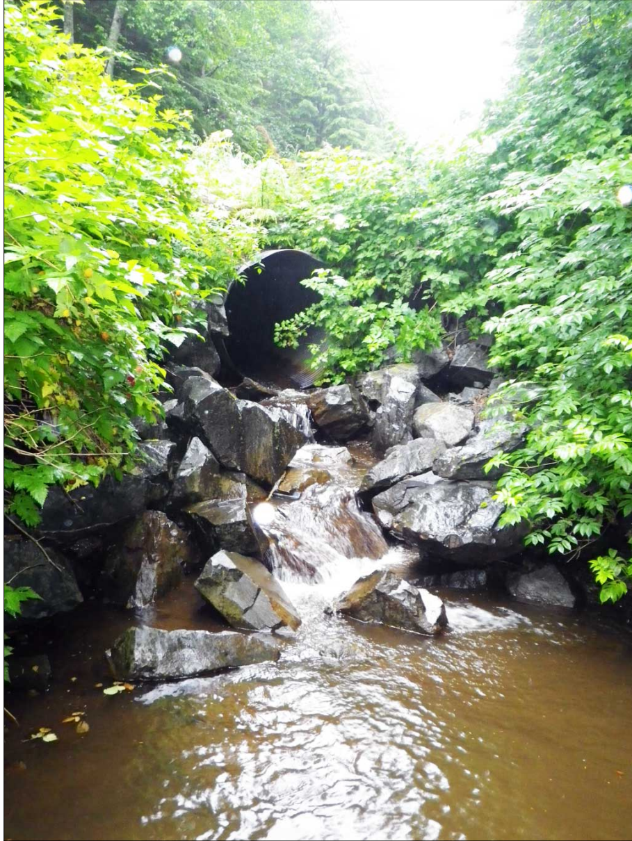
Figure 29.—Site #10303040 on Blueberry Road in Sitka, showing a Red outfall over riprap.
