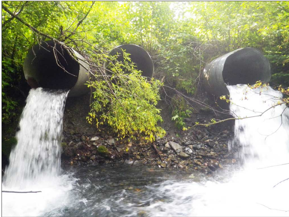
Figure 22.—Site #103022829 culverts on Kelsall Road north of Haines. All culverts perched over 5 feet, with Red gradients and Red constriction. Below this site, the stream is cataloged for coho rearing and pink spawning.
