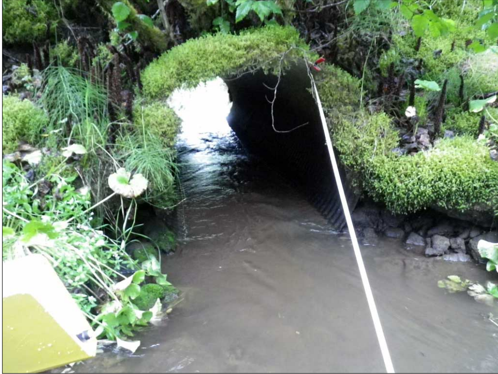
Figure 19.—Site #10302255 in Gustavus showing an undersized culvert with a constriction ratio of 0.40 on a private driveway off Mountain View Road.
