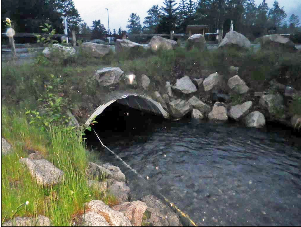
Figure 30.—Site #10302949 with an undersized culvert on Pullen Creek crossing the White Pass and Yukon Route railroad in Skagway.
