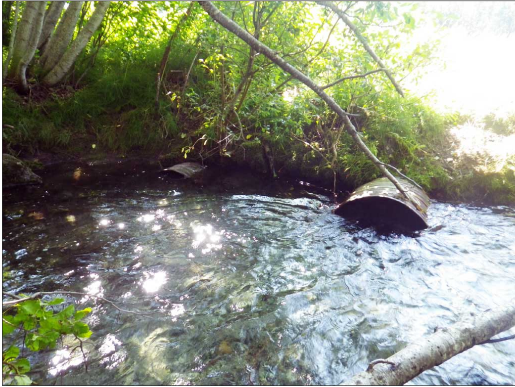
Figure 23.—Site #10302913 undersized culverts on Ten Mile Creek off the Haines Highway.
