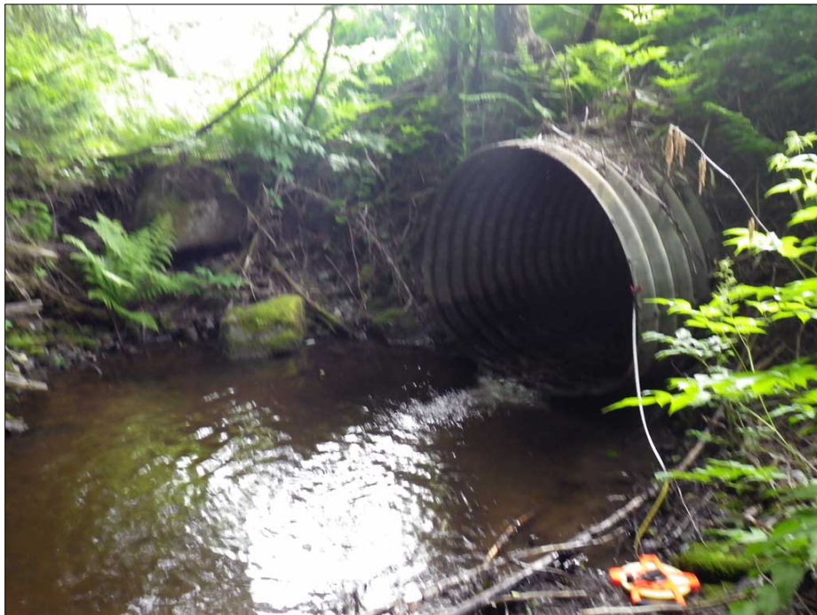
Figure 25.—Site #10302165 culvert on Hendrickson Creek on the North Douglas Highway. Culvert is a gradient barrier and has a Gray constriction ration and outfall height. Creek is cataloged for coho and pink salmon, Dolly Varden, and cutthroat trout.
