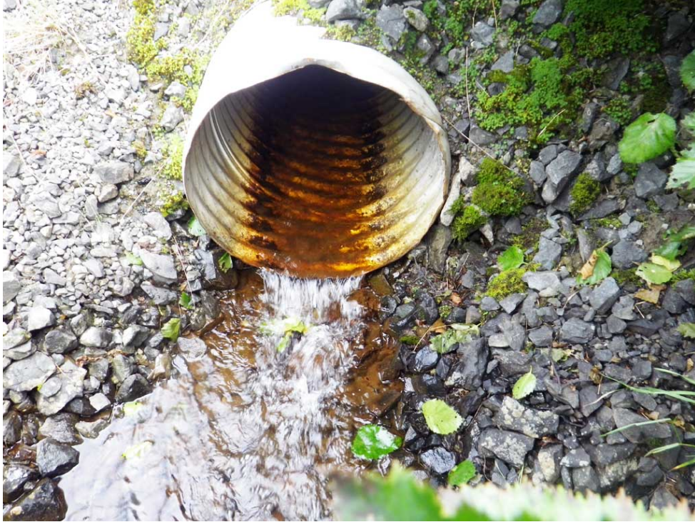
Figure 43.–Site 30103460, outlet of C1 showing outfall.
