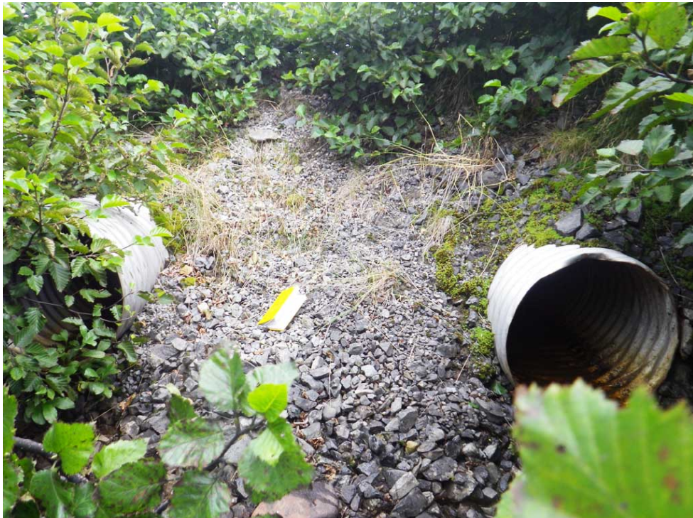
Figure 42.—Site 30103460, culvert outlets.
