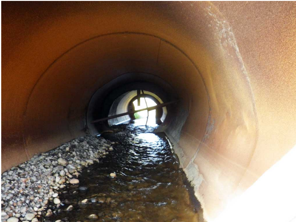
Figure 21.—Site 30103337, looking upstream inside culvert from outlet.
