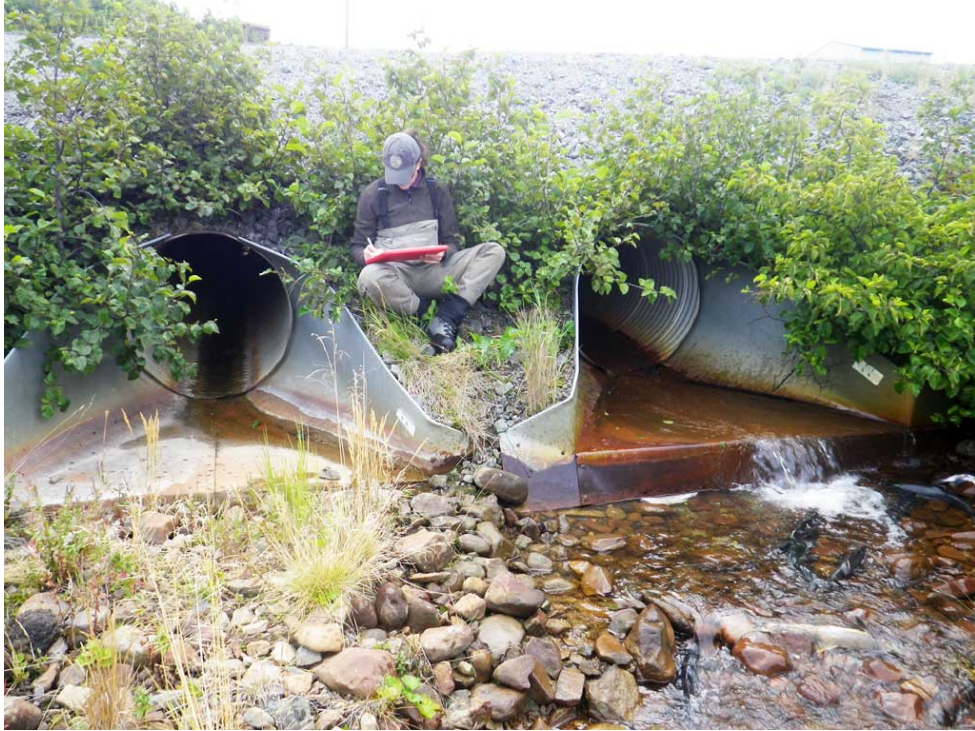
Figure 38.—Site 30103461, outlets showing outfall.
