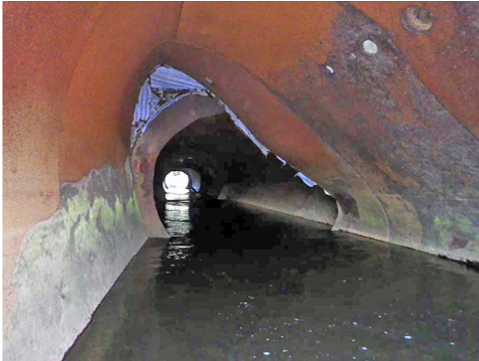
Figure 7.—Site 30103336, internal view of culvert looking upstream from outlet and showing the internal connection between tank sections and the created baffling.
