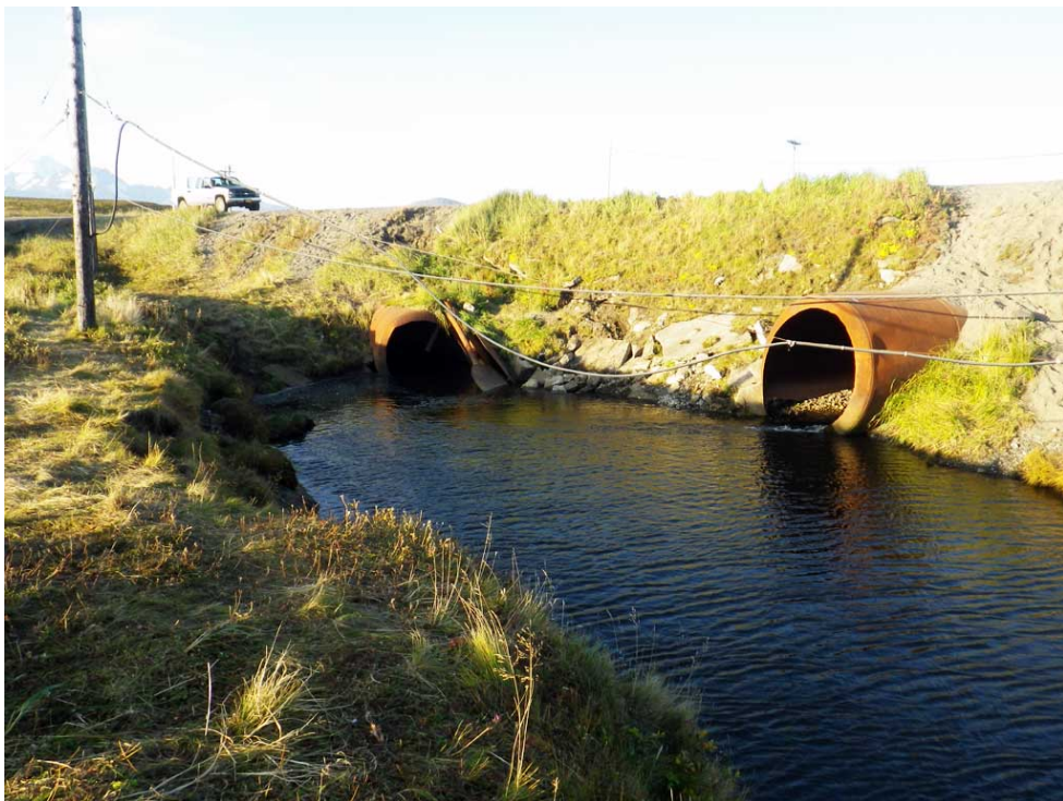
Figure 18.—Outlets of site 30103336 (left) and 30103337 (right)
