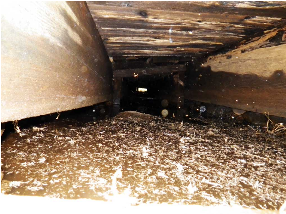
Figure 13.—Site 30103339, looking upstream inside the culvert from outlet.
