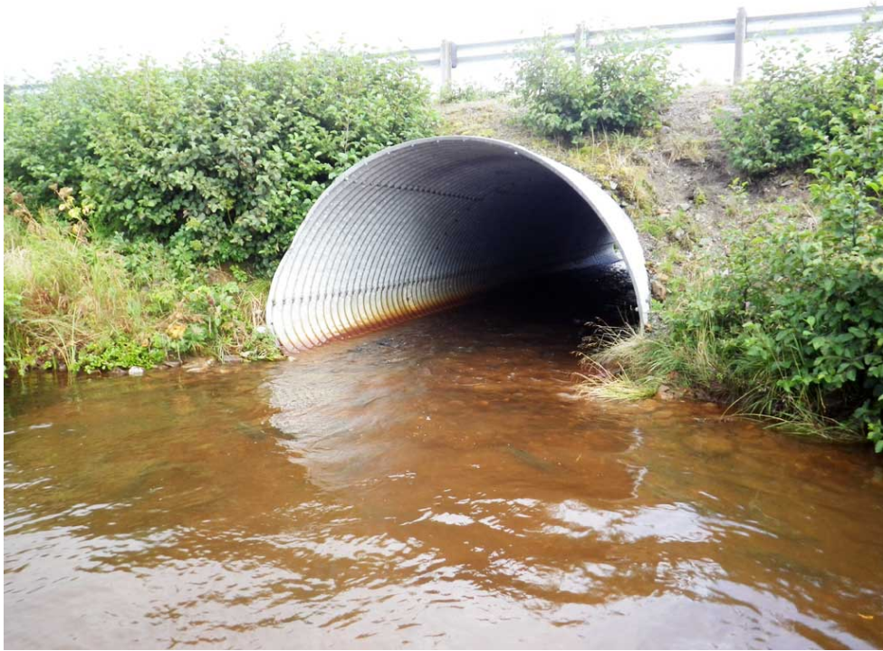
Figure 32.–Site 30103446, culvert inlet.
