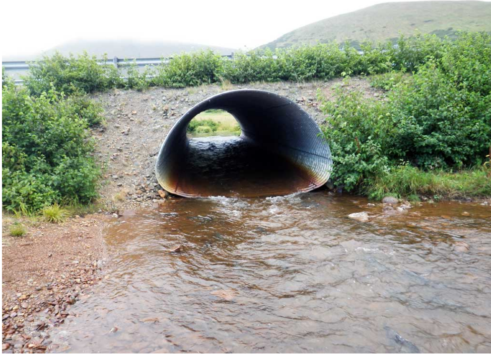
Figure 30.—Site 30103446, culvert outlet showing outfall.
