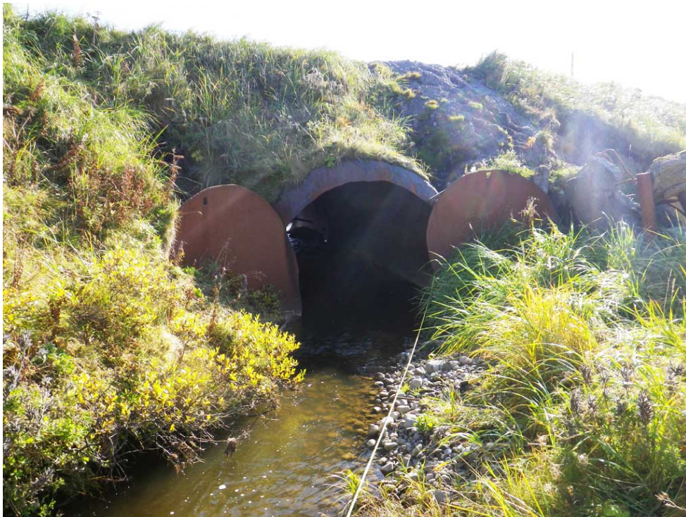
Figure 19.—Site 30103337, inlet with metal wingwalls.
