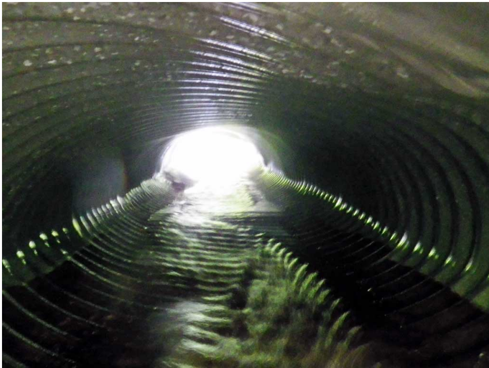
Figure 25.—Site 30103443, looking upstream inside culvert from outlet.
