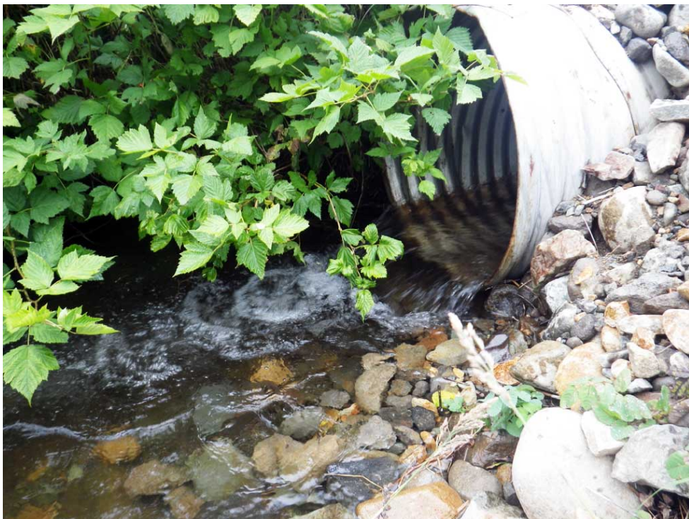
Figure 34.—Site 30103448, culvert outlet showing outfall.
