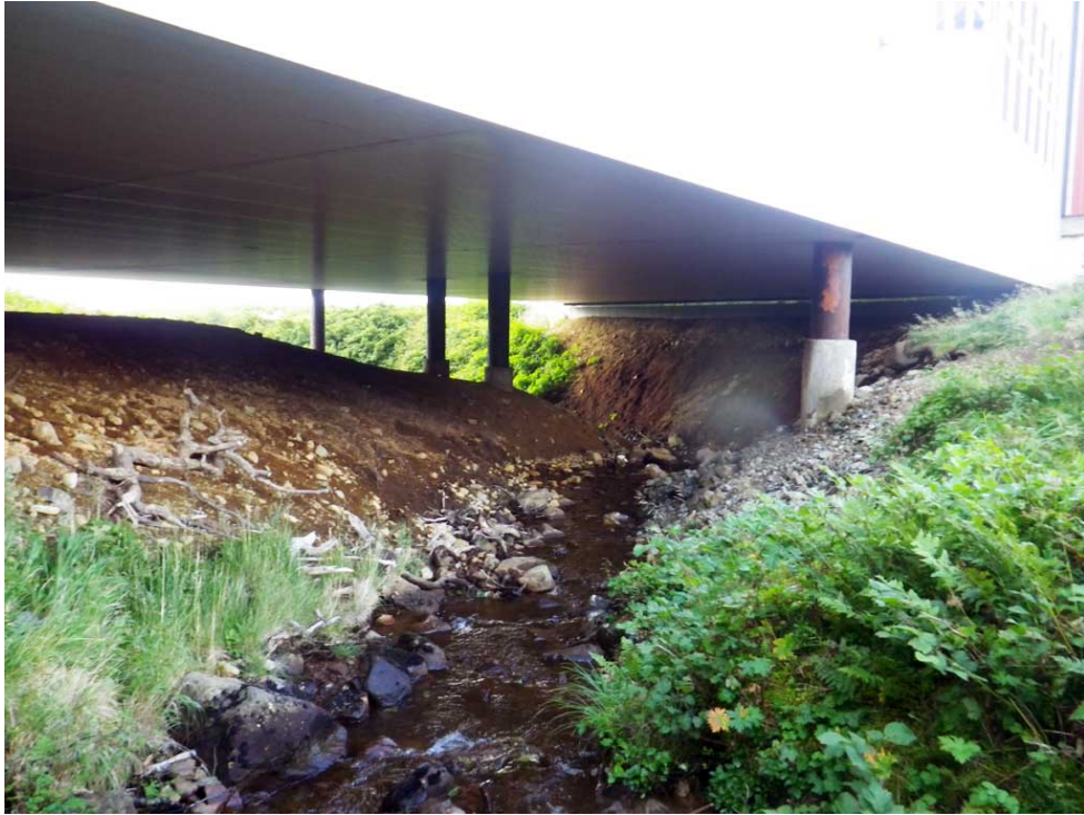
Figure 46.–Site 30103459, 300 feet downstream of culvert showing creek flowing under new King Cove school.
