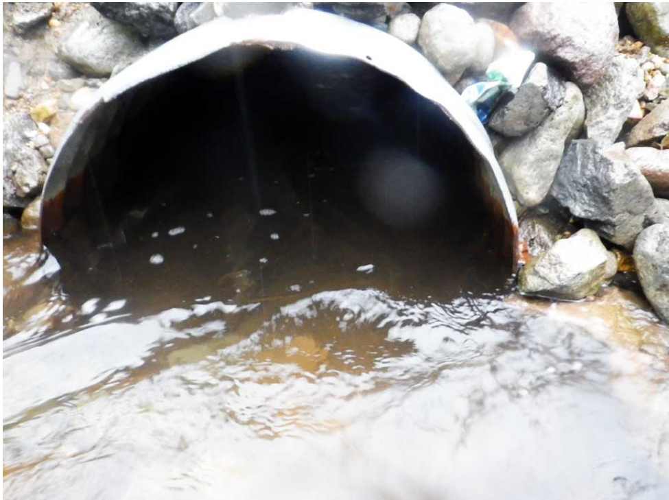
Figure 28.—Site 30103445, culvert outlet from directly downstream.
