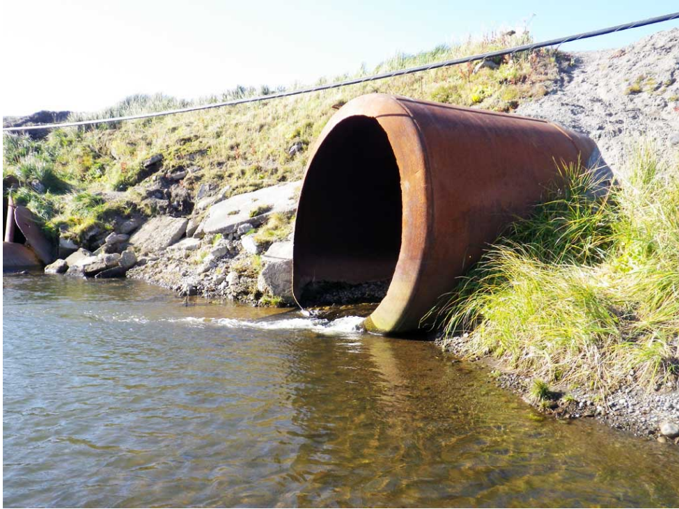
Figure 20.—Site 30103337, outlet showing outfall.
