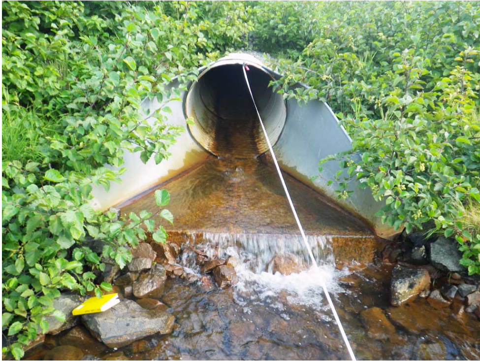
Figure 44.–Site 30103459, flared outlet showing Red outfall.
