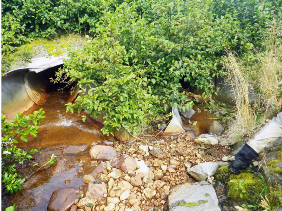
Figure 40.–Site 30103461 culvert inlets.
