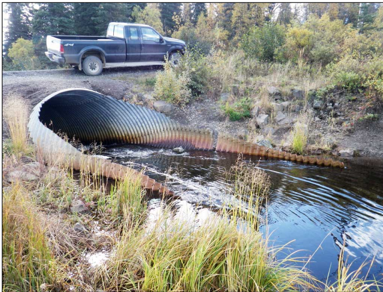
Figure 10.—Site #30303073 Squaw Creek at Lupine Road, Dillingham showing frost heave that has raised the inlet of the culvert several feet causing ponding upstream and a fish passage barrier inside the culvert.
