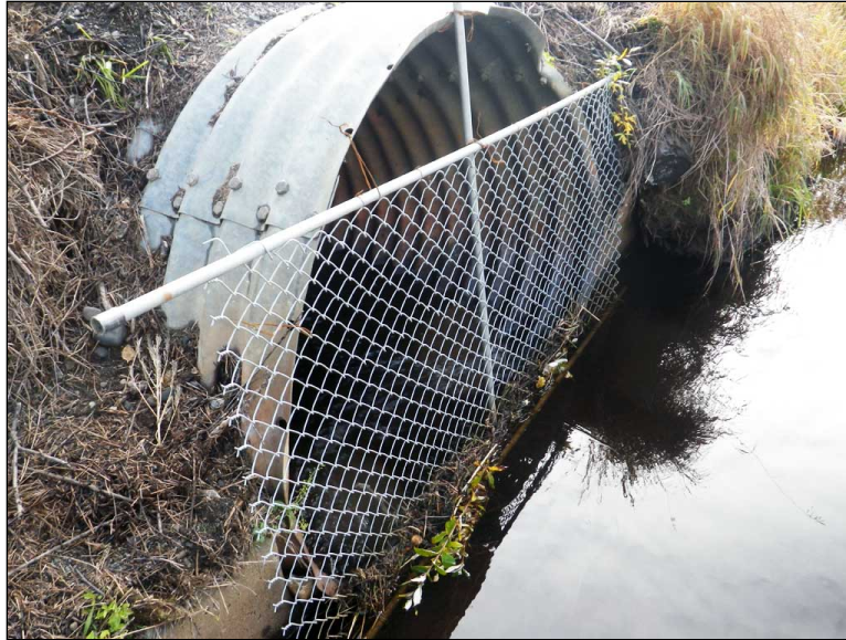
Figure 11.—Site #30303078 showing a chainlink fence preventing fish passage on the South Fork of Squaw Creek, Dillingham.
