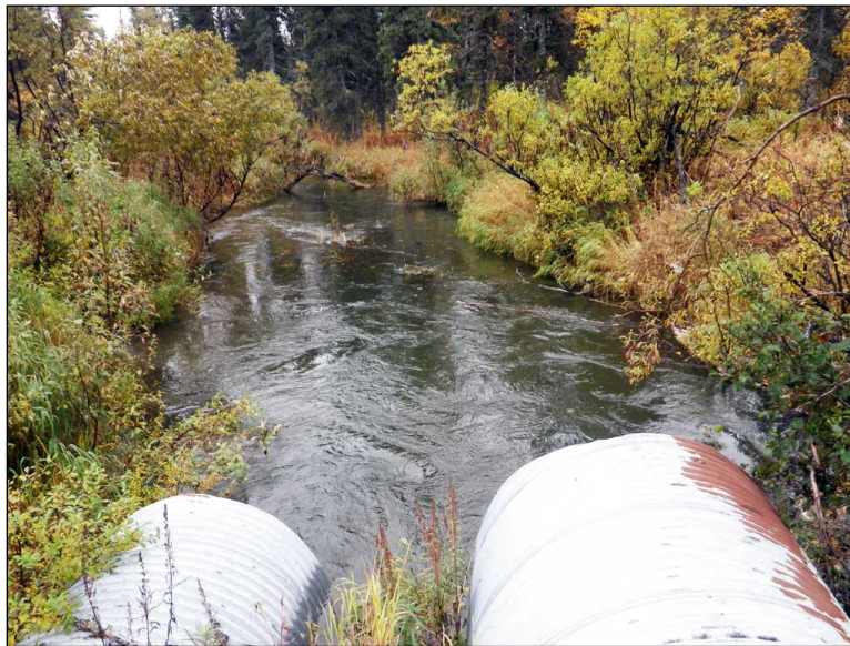
Figure 8.—Site #30303067 showing undersized culverts on a tributary to the Snake River, Dillingham.
