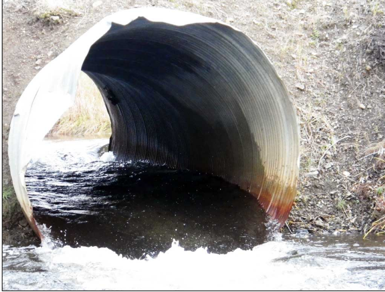
Figure 9.—Site #30303068, an undersized culvert on an unnamed Snake River tributary, Dillingham.
