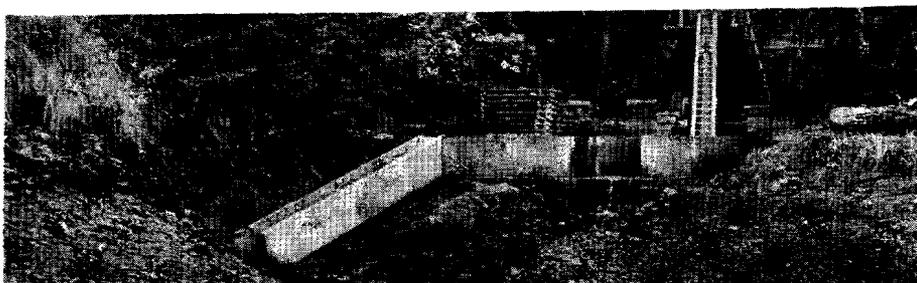
**This steep-pass fishway, result of a development study, will allow salmon to get around a previously insurmountable barrier. Stream was diverted to make this photograph.**
