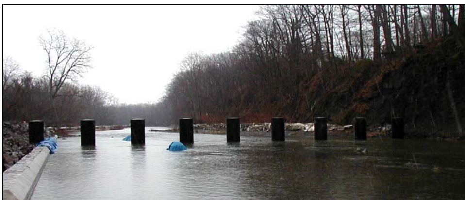
Figure 6. Cazenovia Creek ICS, January 2006, looking upstream. A concrete toe holds riprap along the right bank to prevent scour by floodplain flow returning to the main channel.
