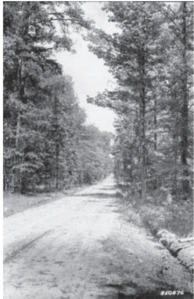
Figure 1— FS Photo 350876. Caption: “Typical 20-foot Forest Service road constructed with CWA hand labor. Road to be graveled and used for utilization of forest products as well as for protection and administration. Road #4 looking east from intersection of roads #4 and #6.” 23 July 1937, Crossett Experimental Forest, Ashley County, Arkansas. (Photo courtesy of U.S. Forest Service, Southern Research Station)
