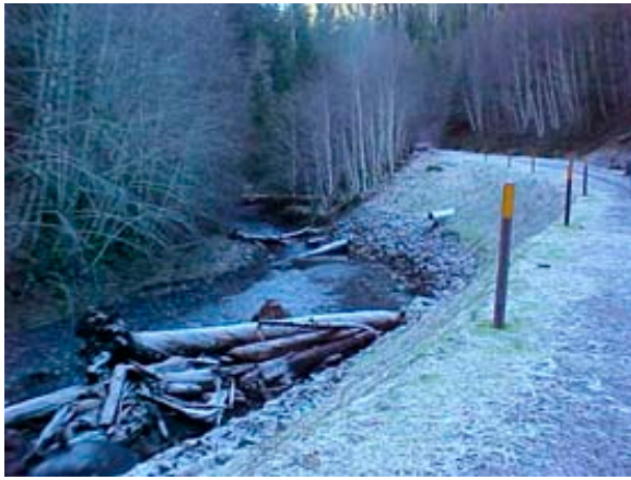
Figure 8: Walter Creek Revetment, Rd 2350 milepost 9.95 - photo of completed project.
