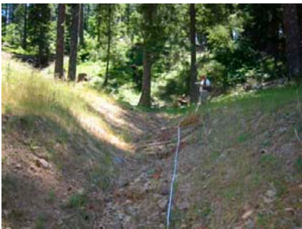
Photo 6: Typical small to moderate size stream crossing excavation - Road 2N14H.
