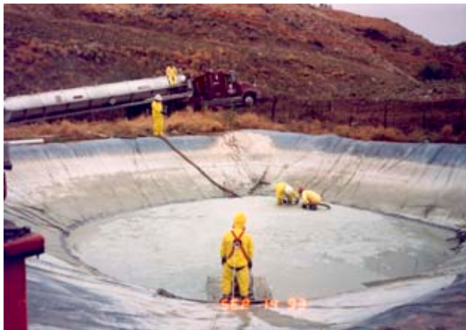
Figure 4. Following reduction of cyanide concentrations the sludges were transported by a licensed Hazmat contractor to the TSD in September 1993.
