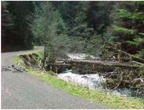
Figure 1. An example of simple encroachment: Site assessment may be limited to the area at and immediately adjacent to the site. Design solutions may be limited to the immediate washout area.
