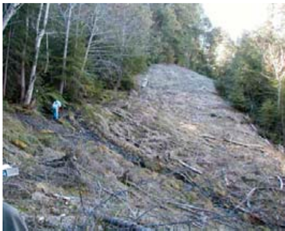
Photo 8: Outsloping associated with unstable roadbed.
