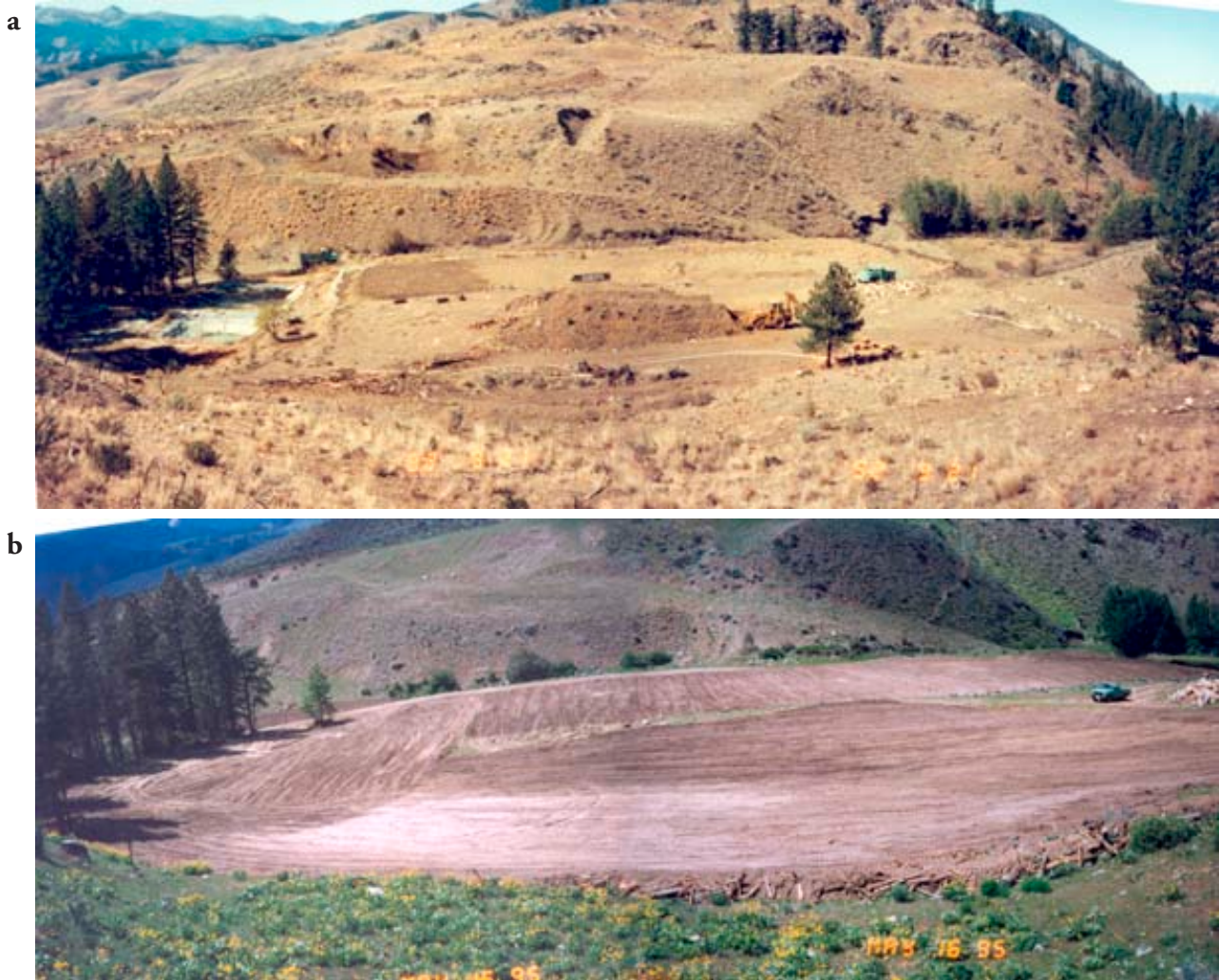
Figure 6. Comparison pre-cleanup disturbances (a) and final cap construction (b).
