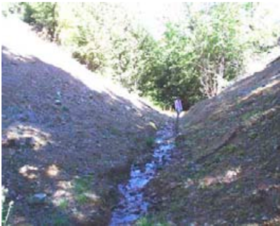
Photo 6: Typical small to moderate size stream crossing excavation - Road 2N14H.
