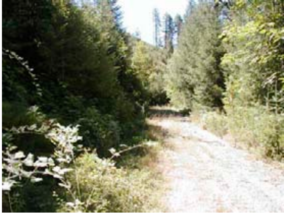
Photo 8: Outsloping associated with unstable roadbed.
