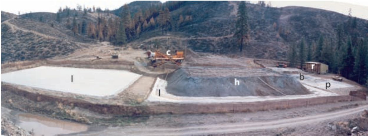
Figure 1. Minnie mine facilities: (h) processed ore heap, (l) pad liners, (p) pregnant process pond, (b) barren process pond, (r) recovery plant. Photograph taken after the 1985 Minnie wildland fire (unrelated to the mine operations).
