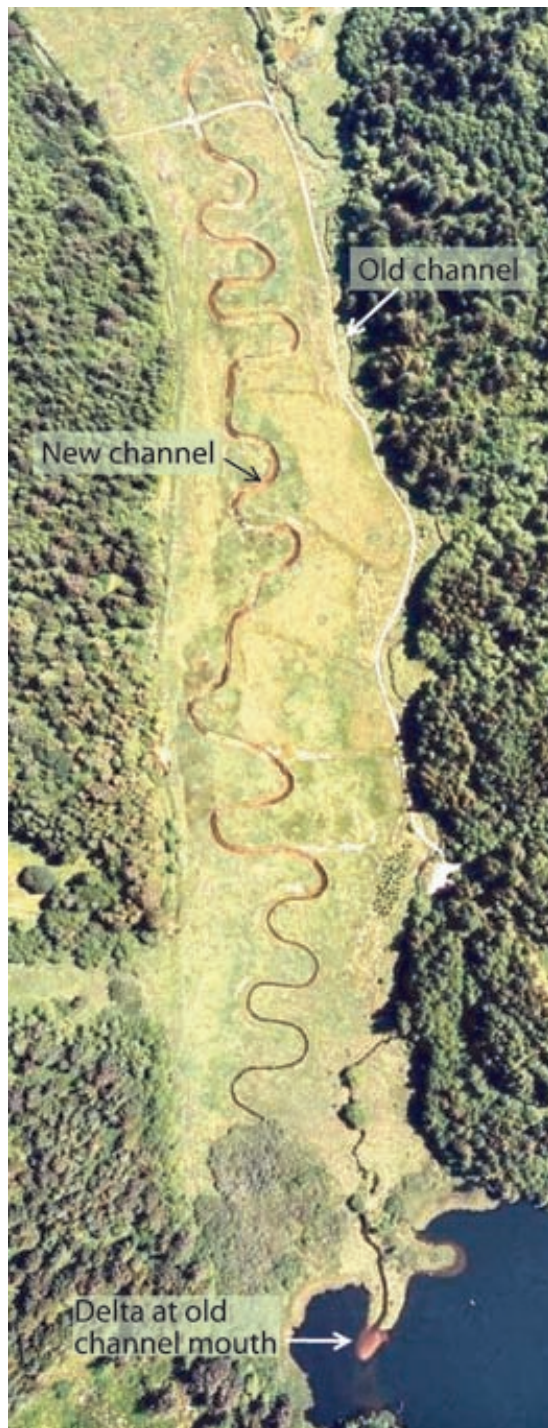
Figure 1: Low-elevation aerial photograph of the new Bailey Creek channel before connection to stream flow. September 2000.
