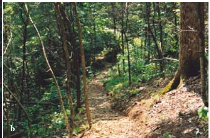
Figure 5. Charles Deam Wilderness Trail, Hoosier National Forest, Indiana. (a) Before, (b) After. Several sections of this popular, heavily used hiking/horseback riding trail were located lower on the slope, with little consideration for cross drainage. This project involved closing and rehabilitating some of the wetter sections, moving the trail farther upslope, adding cross drains, and also surfacing. Photos by Eric Solerno.
