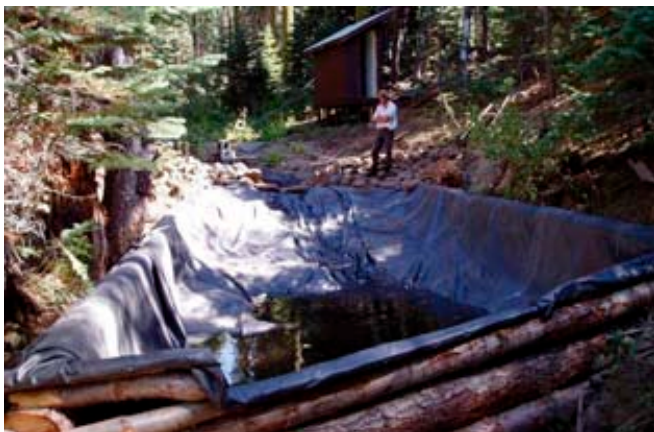
Figure 4. The B204 sediment catchment basin, lined with commercial pond liner, traps sediment behind a 1.2-meter-high log structure. Sediment is removed each fall, weighed wet and subsampled. A dried subsample is analyzed to determine organic and mineral fractions and particle size distribution.
