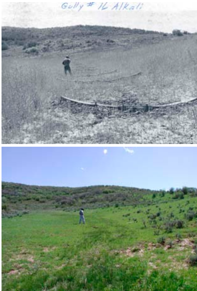
Figure 14. (a) Vegetation-lined waterway No.16 in early 1960s with burlap strips in place to disperse flow. Photo by B. Heede. (b) The same waterway in the early summer of 2004. Photo by C. Hirsch.
