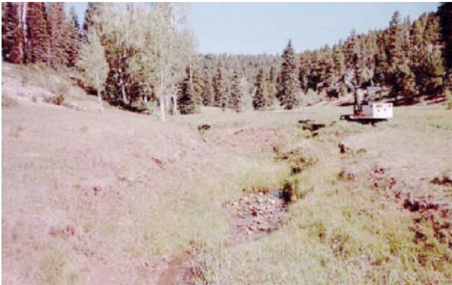
Figure 1: PP #7. Looking upstream on main channel (7/2000)
