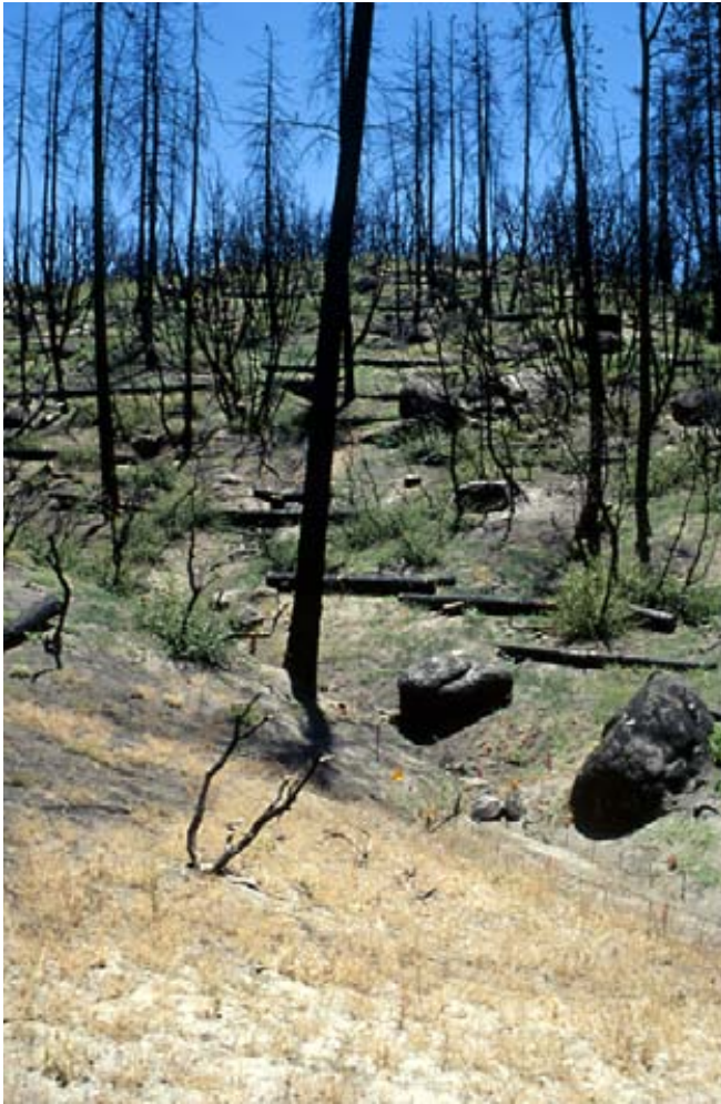
Figure 2. Overlapping network of log erosion barriers (LEBs) on the Mixing Fire site.
