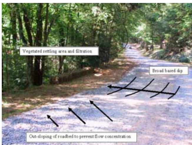
Figure 5: Example of a properly constructed broad based dip from the Conasauga River Large-Scale Watershed Restoration Project, Cohutta Ranger District, Chattahoochee National Forest, USDA Forest Service (photo by M.S. Riedel).
