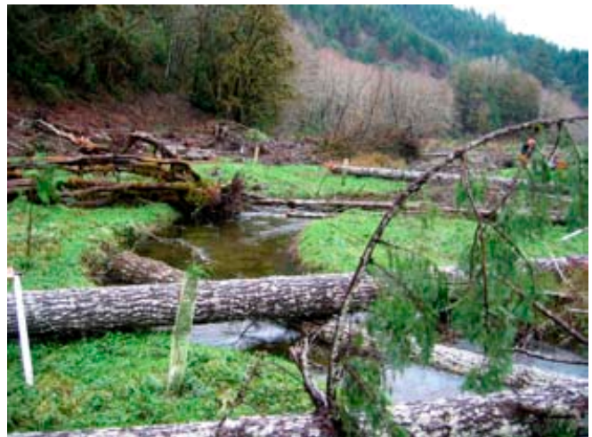
Figure 8. The new Karnowsky Creek channel with large wood added, winter 2003. New conifer seedlings are planted along the bank and protected by plastic tubing.
