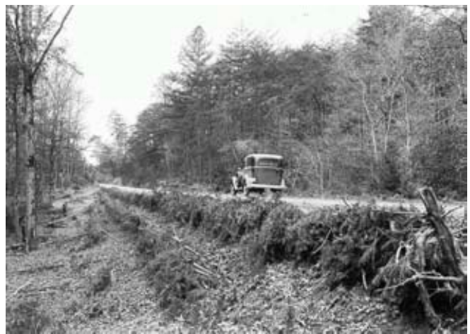
Figure 3: Example of early bioengineering to stabilize a cut slope road embankment (photo by C.R. Hursh).
