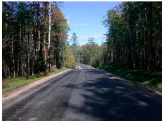
Figure 6. Road improvements on the Huron-Manistee National Forest, Lower Michigan. (a) Before, photo by William Fowler, (b) After, photo by Robert Stuber. Former road was narrow, with native material for road surfacing; drainage structures were undersized with many acting as barriers to aquatic organism passage. Road surfacing was hardened; alignment improved, some of the crossings were elevated; drainage structures were replaced with at least one bridge added; side slopes were stabilized and outlet drains provided to catch and direct runoff. This was a 2-mile long project that occurred over three years.
