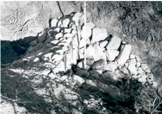
Figure 8. Typical single fence check dam. Photo by B. Heede.
