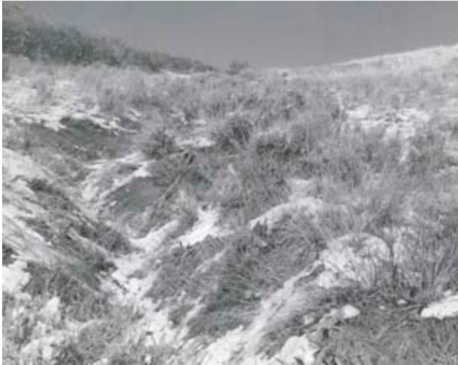
Figure 10. (a) Vegetation lined waterway construction sequence. Original gully configuration. (b) Shaping the new waterway after filling and compacting the old gully. (c) Completed waterway after establishment of vegetation. Note that the new flow line is offset from the original gully location. Photos by B. Heede.
