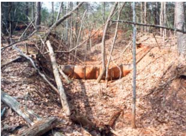
Figure 10. Following autumn leaf fall, indicators of gully activity with respect to sediment delivery disregarding the filter fabric fence are masked to the casual observer.
