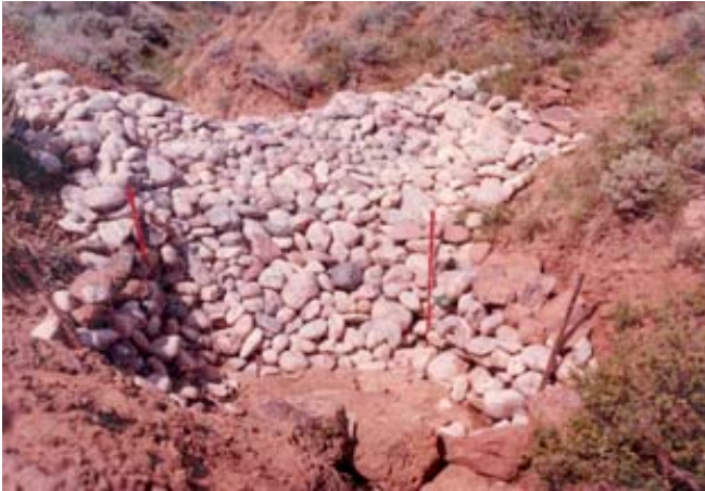
Figure 8. Typical single fence check dam. Photo by B. Heede.
