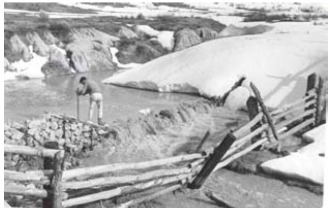
Figure 11. (a) Double fence check dam at the base of the main gully (structure M0) during peak snowmelt runoff in the spring of 1964. Photo by B. Heede. (b) The same double fence check dam during the fall of 2004. Photo by M. Weinhold.
