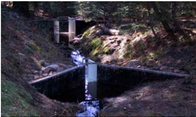
Figure 2. The two-flume design on the B201 stream allows KREW staff to precisely measure a wide range of flows. The 3-inch Parshall Montana flume (foreground) measures most flows, and the 2-foot Parshall Montana flume (background) measures large rain events.
