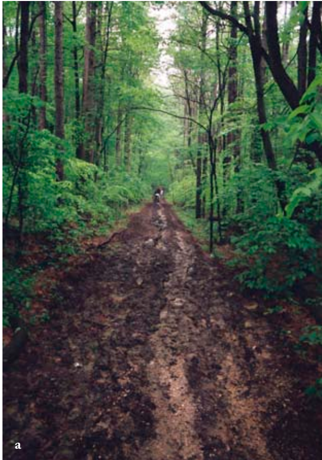
Figure 5. Charles Deam Wilderness Trail, Hoosier National Forest, Indiana. (a) Before, (b) After. Several sections of this popular, heavily used hiking/horseback riding trail were located lower on the slope, with little consideration for cross drainage. This project involved closing and rehabilitating some of the wetter sections, moving the trail farther upslope, adding cross drains, and also surfacing. Photos by Eric Solerno.
