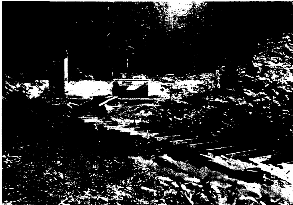
Figure 4.--Intake flume, stilling basin, and outlet to channel showing V-notch weir and gage house.
