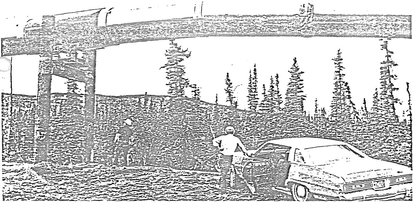
Although not specifically designated as animal crossings, some elevated portions of the trans Alaska pipeline provide adequate clearance for passage of large migrating or roaming animals. There are about 360 such sites along the 800-mile line.
