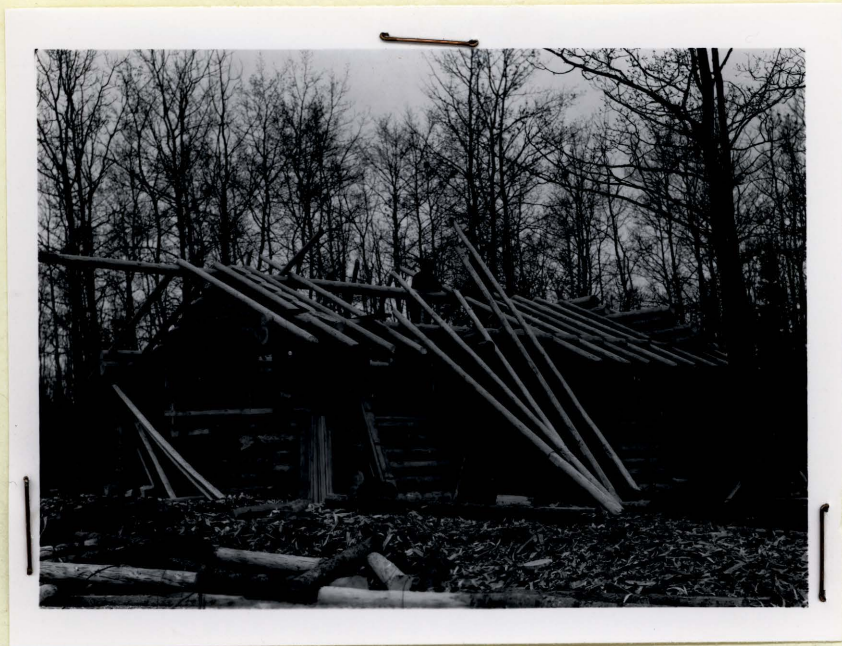
PUTTING ON RAFTERS
