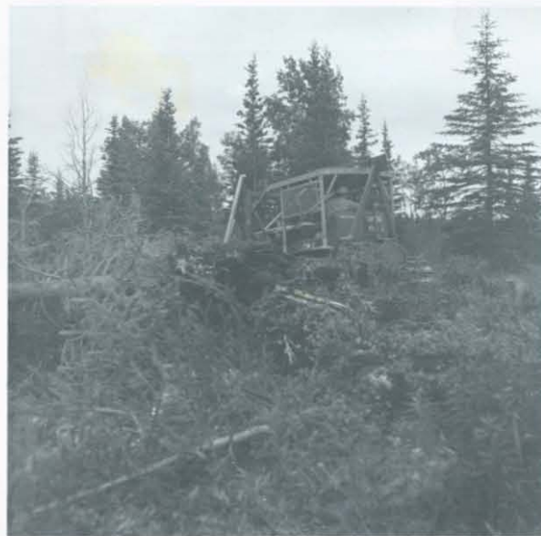
Figure 4. Blade cuts tree stump at ground level.
