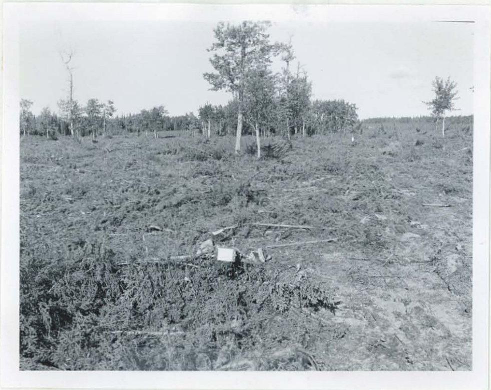
Figure 10. Forage experimental plot #7 after treatment with Crossville plow.
