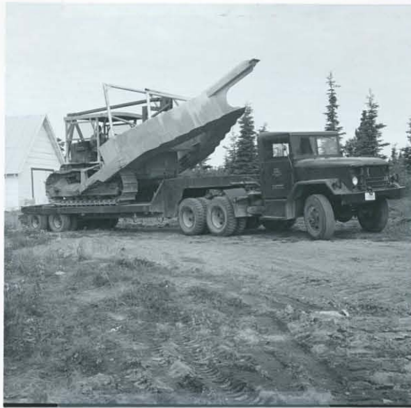
Figure 1. Loading D-7 with Crossville land clearing blade on BSW lowboy.
