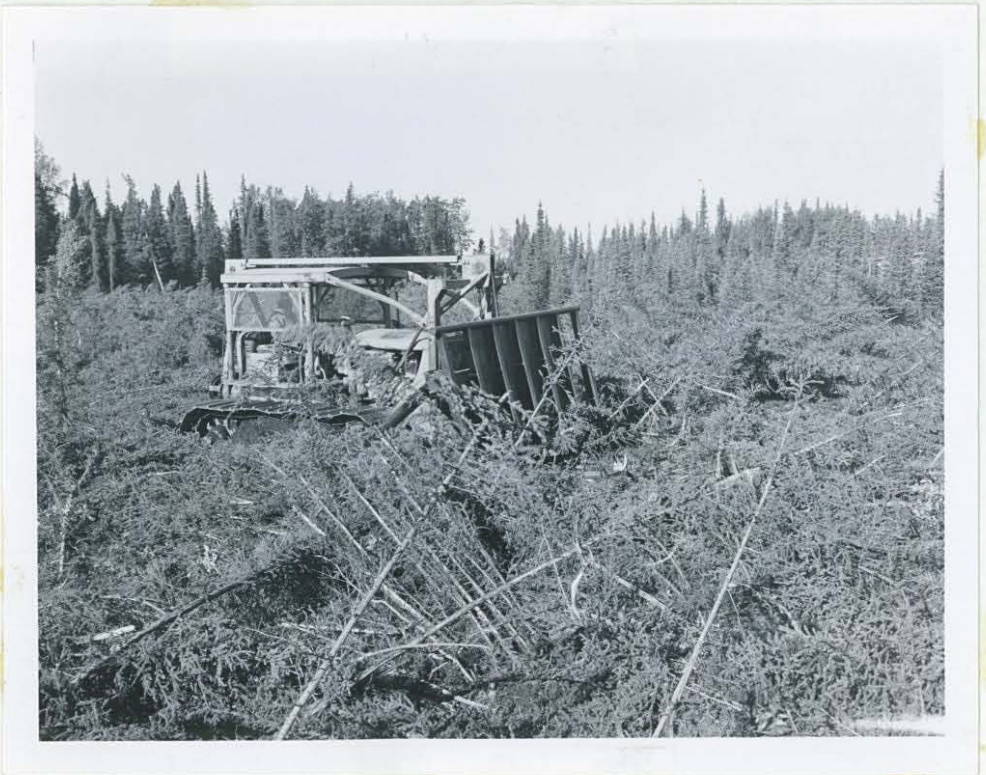
Figure 9. D-7 tractor in action using Crossville rake.
