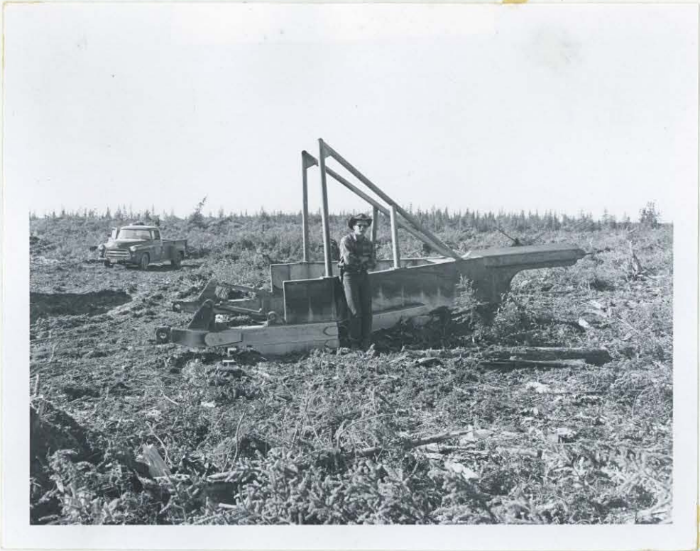
Figure 8. Crossville land clearing plow.
