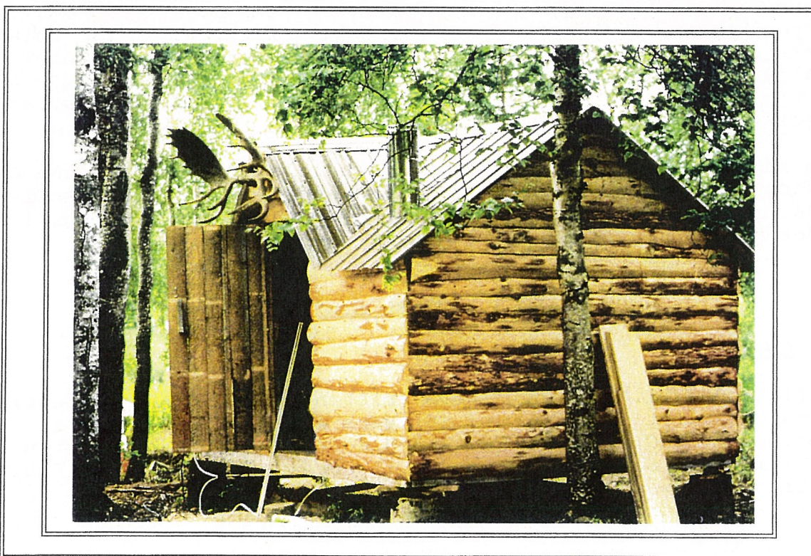
more easily maintained, not to mention, nice looking structure (KE 7/94).
