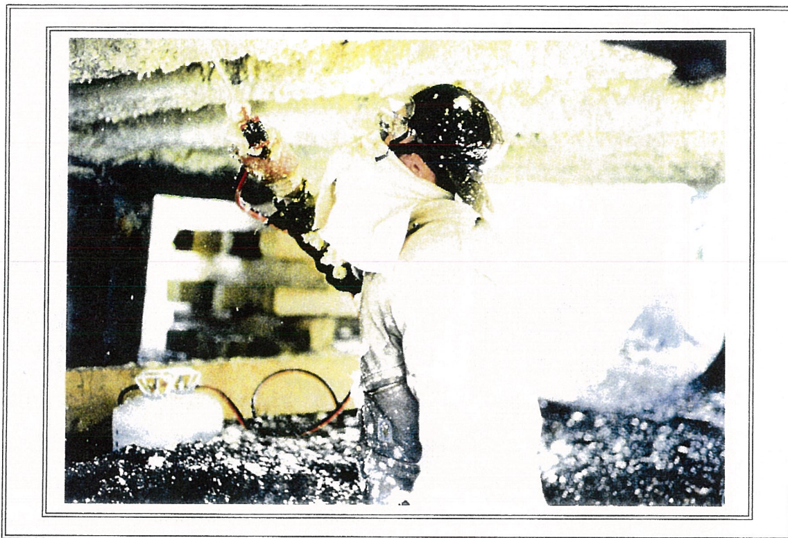
Small Engine Mechanic (SEM) Reid uses foam to insulate the floor of the newly raised cabin (KE 8/94).
