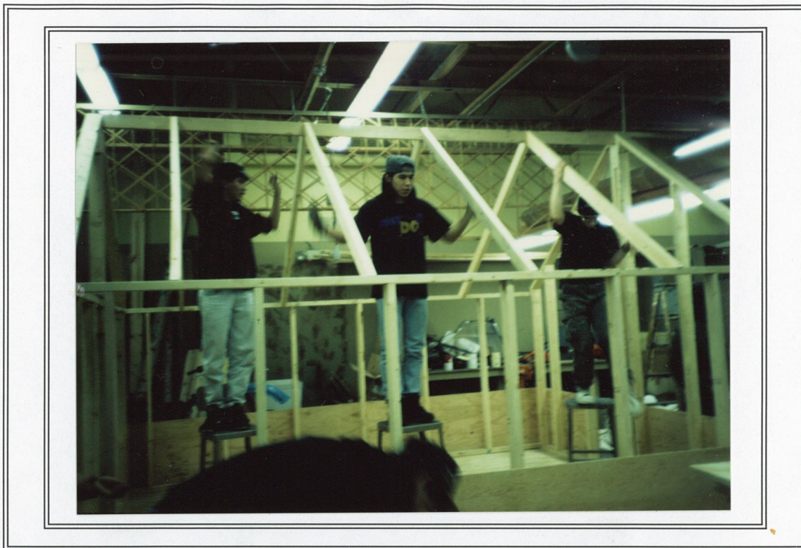
McGrath/Shageluk Village Living Skills students designed and prefabricated the tent frames that were to be used during the Refuge Environmental Education Camp. (BS 2/93)
