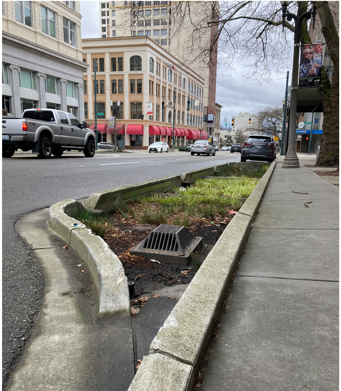
Figure 1: Catch basin grates in Tacoma, Washington.
