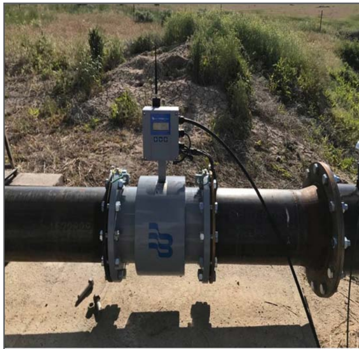
Figure 11: Telemetered Data Acquisition Installation
