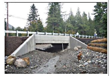
The new crossing is a 27 ft (8.23 m) wide concrete box structure that provides access to 2.4 mi (3.9 km) of potential habitat for chum and coho salmon, steelhead, sea run cutthroat, resident and bull trout.
