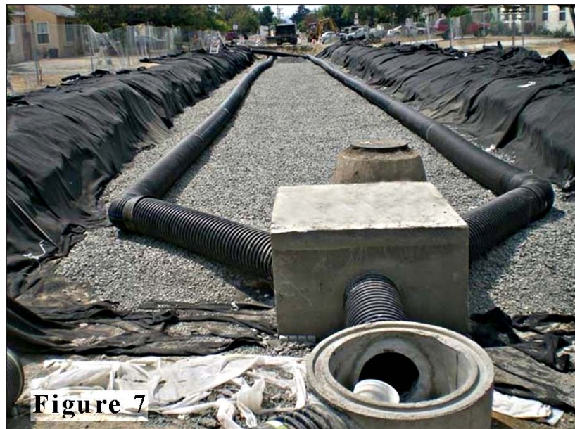
Figure 7 – Elmer Avenue Infiltration Gallery under Construction
