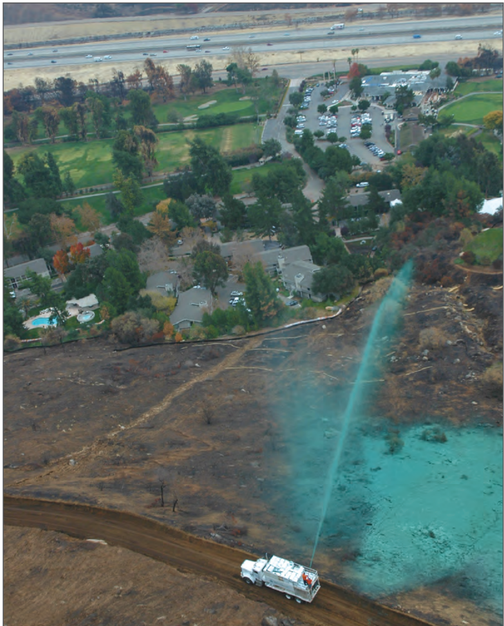
Figure 5. Aerial photo of the application of an hydraulic matrix following the 2007 Witch Creek Fire in San Diego, CA 2007.
