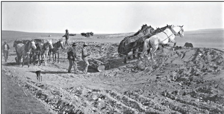
"Fresno" scrapers being used for irrigation canal construction circa 1910 Source: Rowley, The Bureau of Reclamation: Origins and Growth to 1945 (Reclamation 2006)
