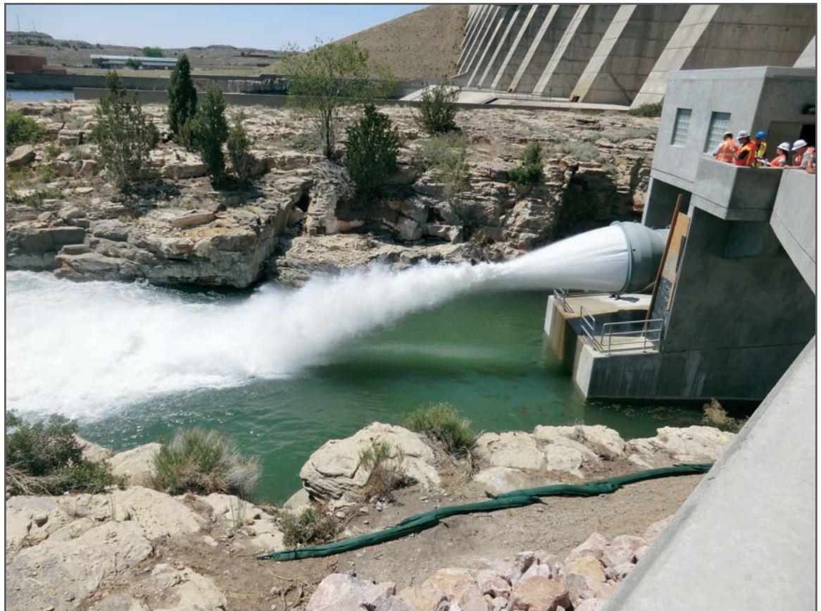
Dam Connection: The newly constructed connection to Pueblo Dam, a federal facility, was completed and successfully tested in the summer of 2012. This connection serves as the origination point of the SDS project with valves to control releases to the Arkansas River and raw water delivered north through the pipeline.
