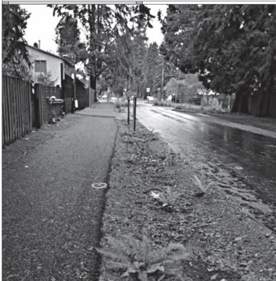
Shoreline Residential Street with Porous Asphalt Walkway and Bioinfiltration Planting Area — SvR Design Company Photo
