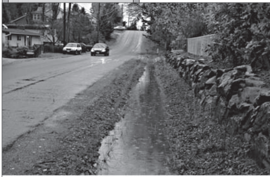
Shoreline Residential Street with Bioretention Swale — SvR Design Co. Photo
