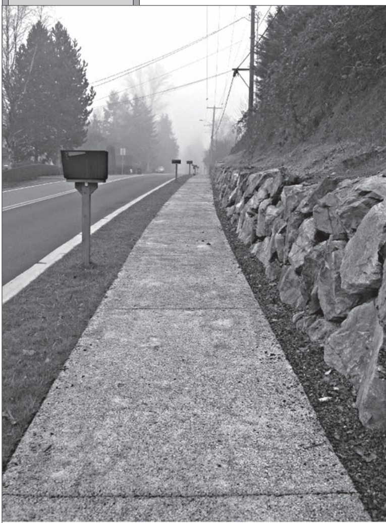
Kirkland Street with pervious concrete sidewalk — SxR Design Co. Photo
