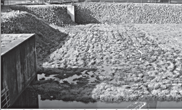
Photo 2: Parallel Bioswale showing preferential pathways
