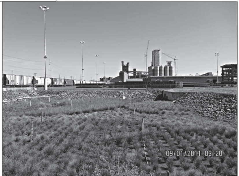
Photo 8: Conversion of Existing Bioswale to a Bioretention System Completed in 2009
