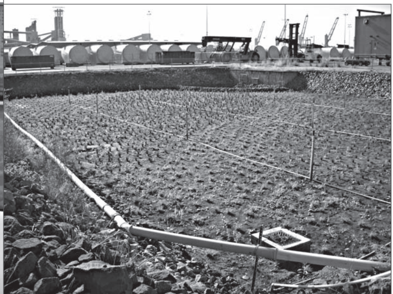
Photo 6: Installation, following replacement of plants &amp; improper media
