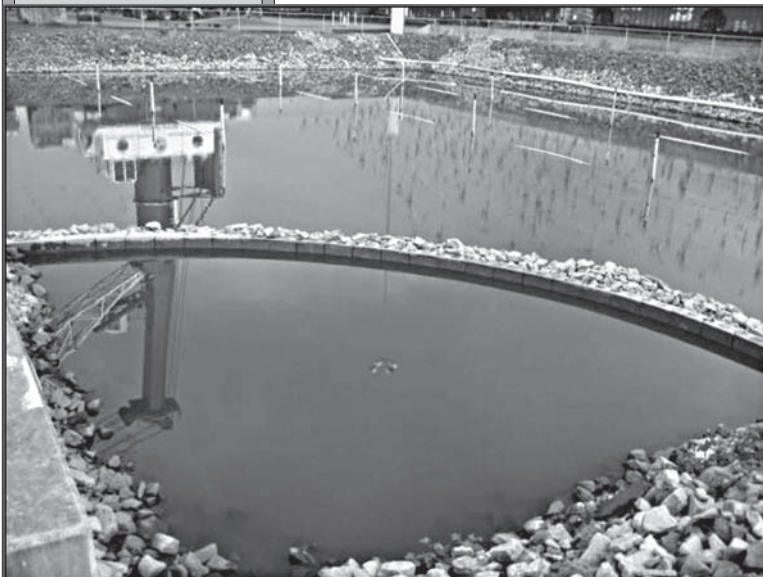
Photo 3: Initial Bioretention System showing poor infiltration due to improper aggregate/compost mix
