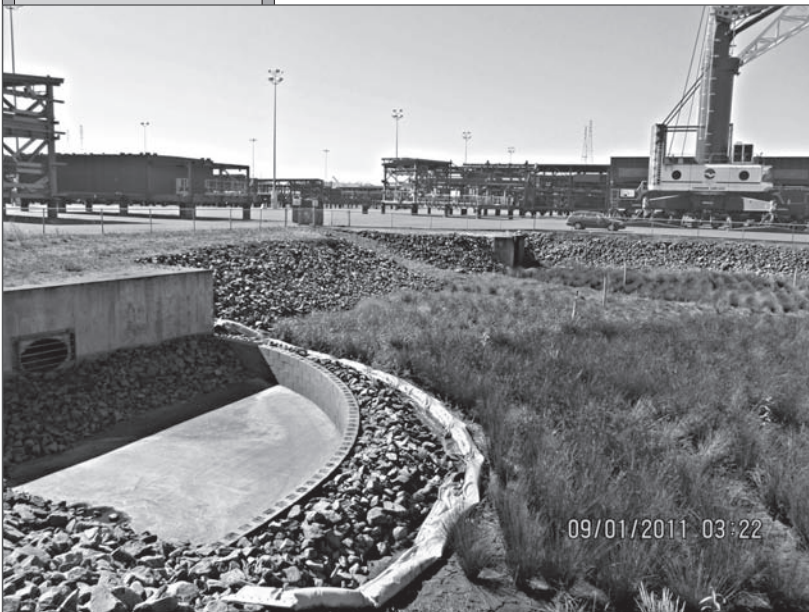
Photo 7: Conversion of Existing Bioswale to a Bioretention System Completed in 2009
