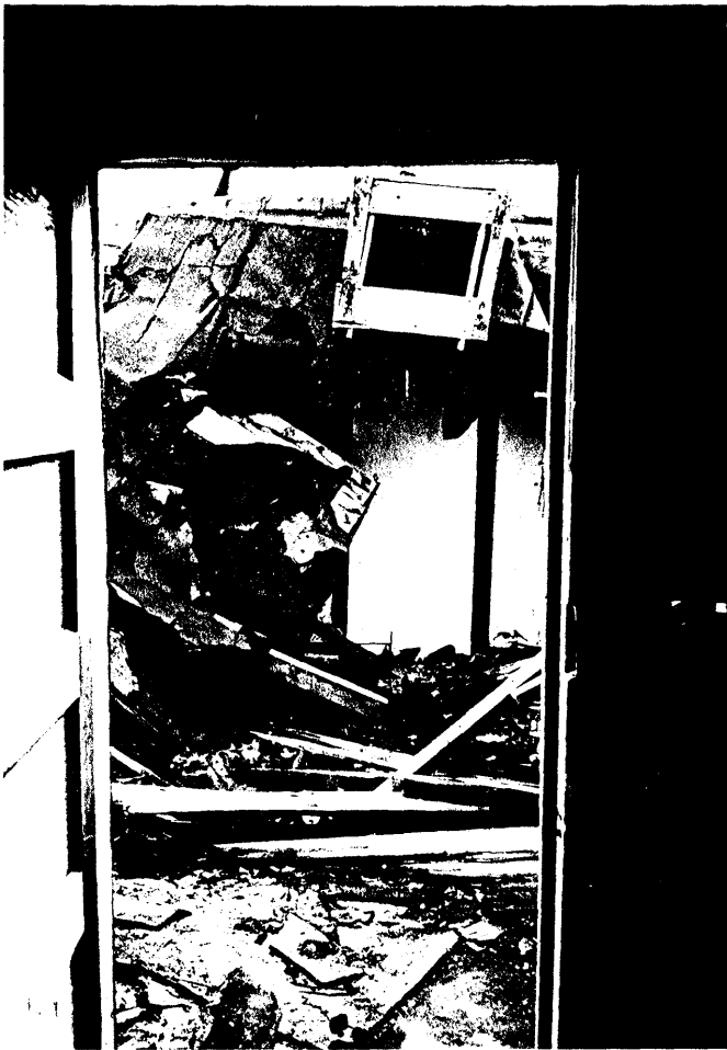
Photo 8: Mess Hall Addition
