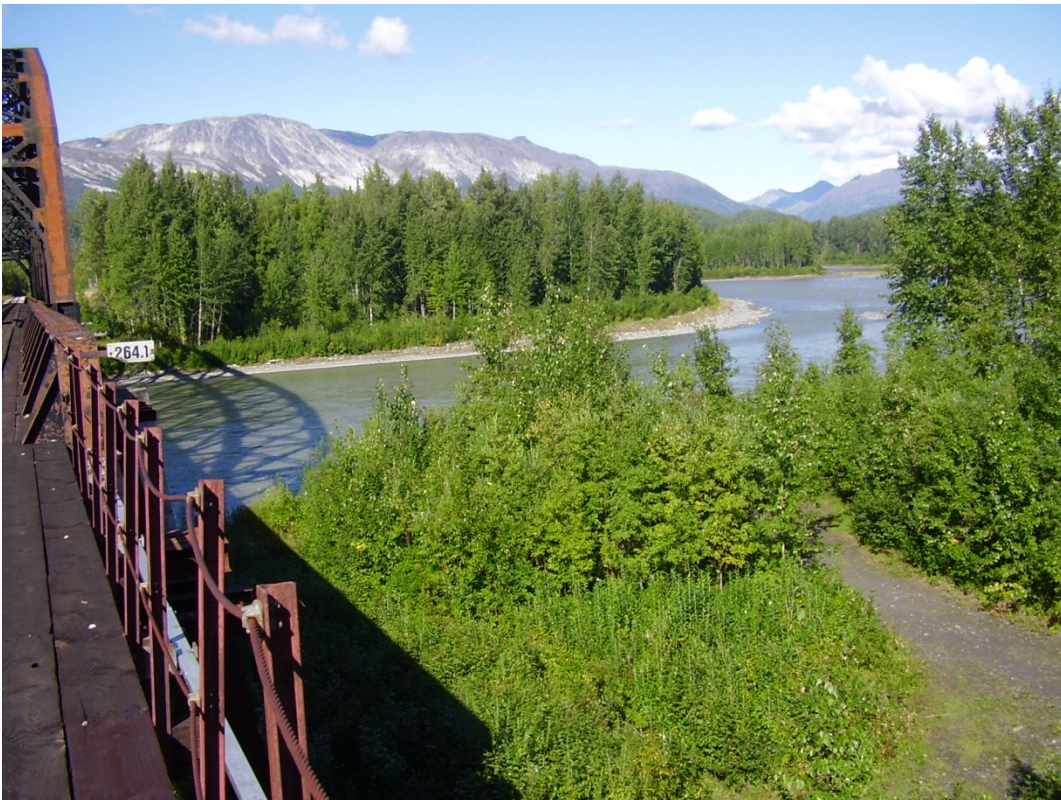
Railroad bridge crossing Susitna River near Community of Gold Creek, looking northeast
