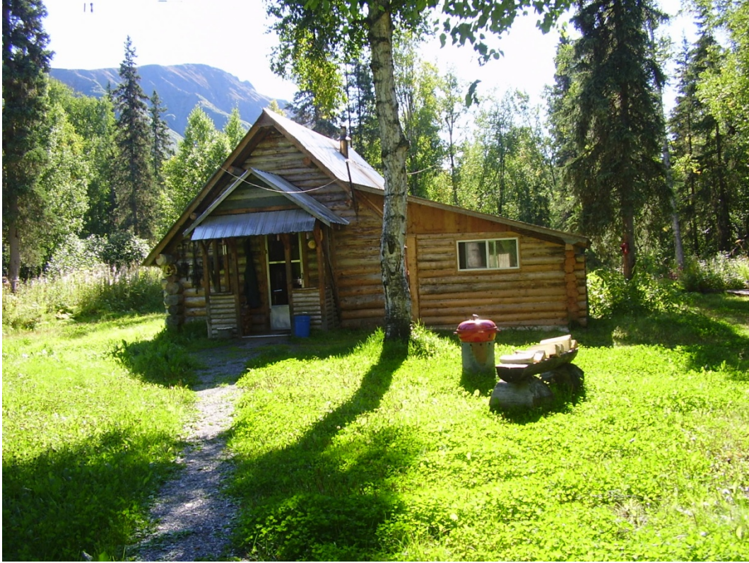
Cabin in Community of Gold Creek
