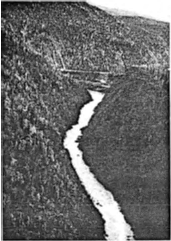
PHOTO E1.8.1: DEVIL CANYON RAPIDS LOOKING UPSTREAM TO DEVIL CANYON DAMSITE
