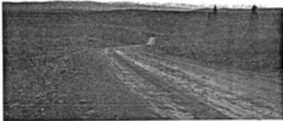
PHOTO E4.8.3: DENALI HIGHWAY (LOOKING SOUTHEAST) NEAR PROPOSED ACCESS ROAD. JUNCTION. THIS IS A TYPICAL COMPACTED GRAVEL ROAD AND IS SIMILAR TO THE PROPOSED ACCESS ROAD
