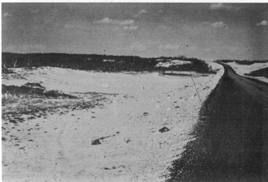
Fig. 1.—A road recently constructed through reindeer range in Finnmark, Norway. Excessive destruction of vegetation has resulted from careless construction practices. The loss to reindeer range in the area has been substantial.
