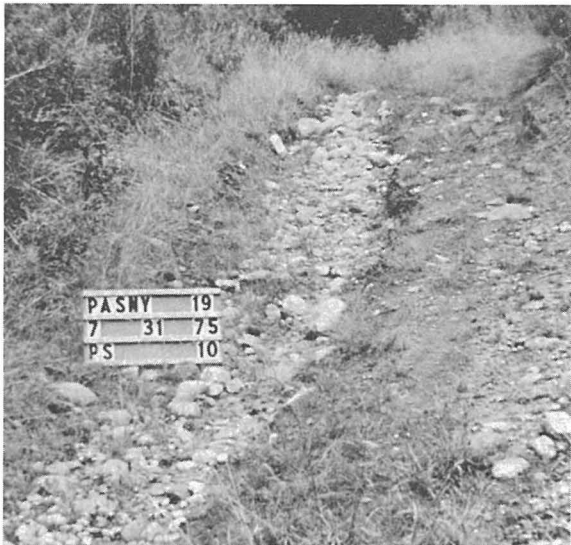
FIG. 19.1.3. Severe gully erosion on access road on ROW, in summer, 1975 (Photo Station 10).
