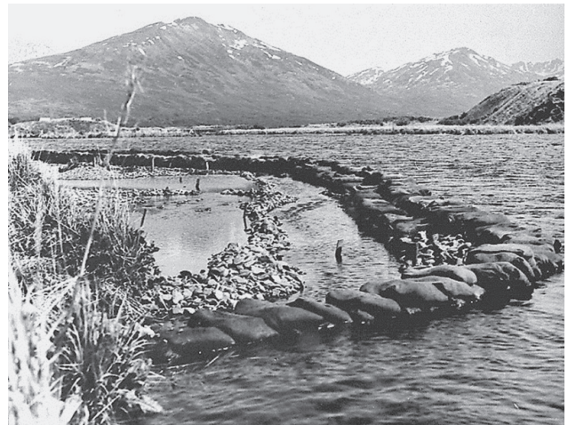
Coffer dam for construction of a two-way permanent salmon counting weir, upper Karluk River, June 1949. (Richard F. Shuman, Auke Bay Laboratory, Auke Bay, AK)
