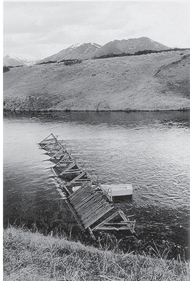
Dolly Varden temporary angled weir, Karluk River Portage, May 1941. (Allan C. DeLacy, from Catherine J. DeLacy, Seattle, WA)
