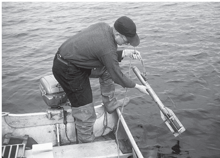
Fisheries Research Institute biologist using a bathythermograph, Karluk Lake, 1952. (Charles E. Walker, Sechelt, BC)
