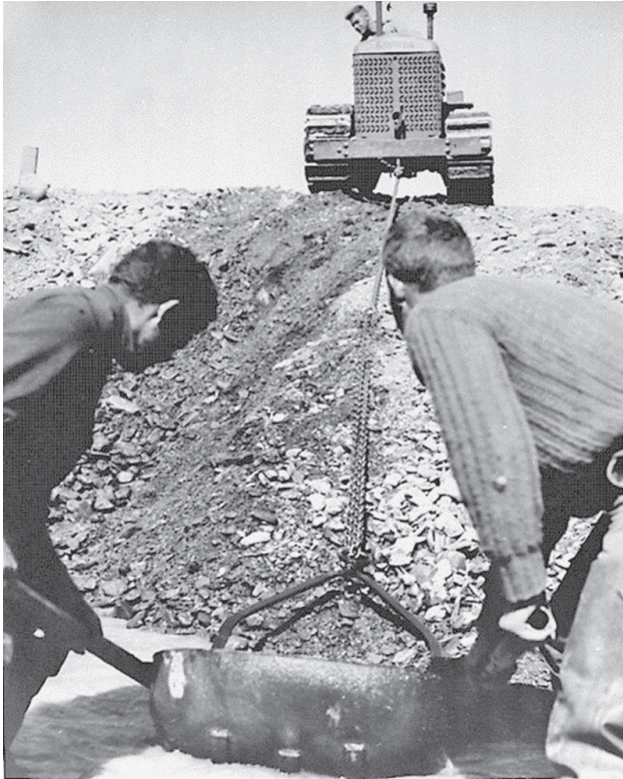
Using a slip scraper and Cletrac tractor to excavate the footing for a two-way weir, upper Karluk River, June 1949. (Richard F. Shuman, Auke Bay Laboratory, Auke Bay, AK)
