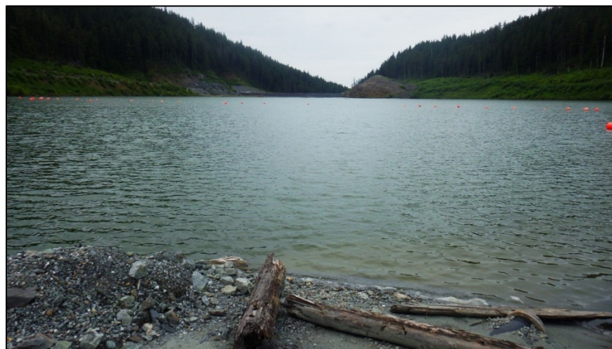
Figure 8.—Tailings treatment facility.
