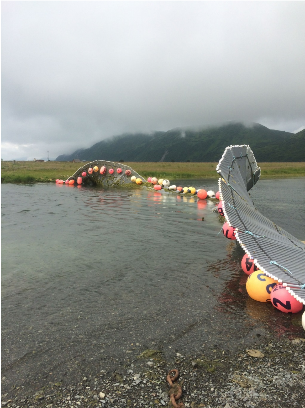
Figure 12.—Pasagshak River floating weir flipped upstream after large upstream current.
