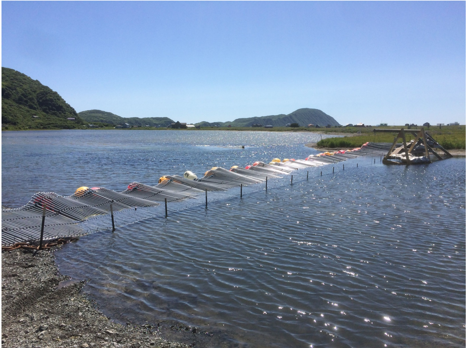
Figure 5.—Pasagshak River floating weir, 2016.
