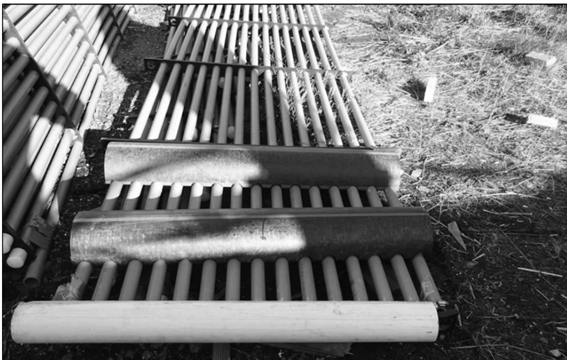
Figure 3.—Example of Unalakleet River weir boat gate panel with HDPE pipe sections to safeguard PVC weir pickets against propeller strikes.
