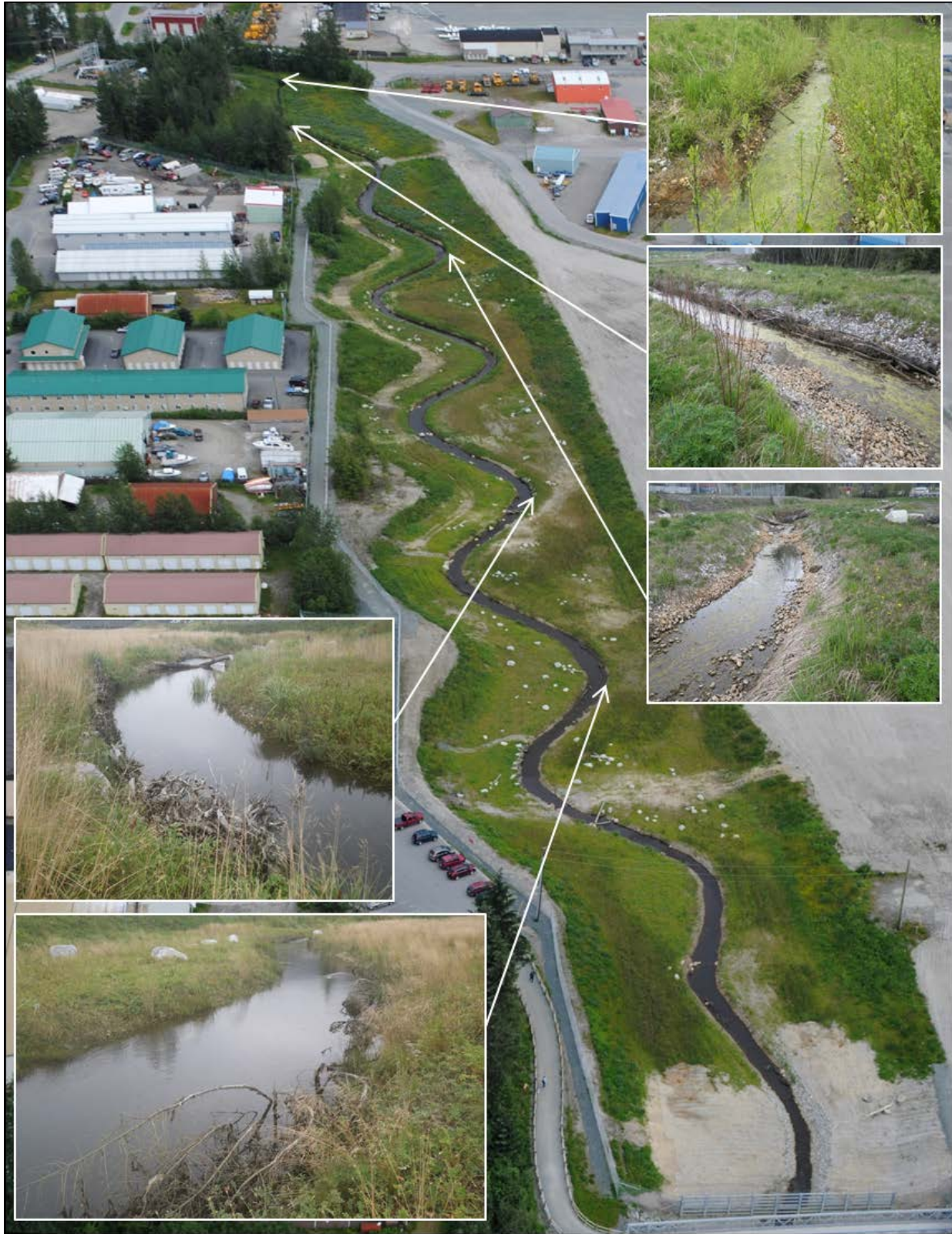
Figure 4.—Realigned channel and instream structures, July 2012.
