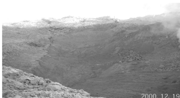
Figure 6. Till blanket placed in the talik.
