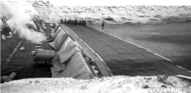
Figure 5. Liner installation during the winter.
