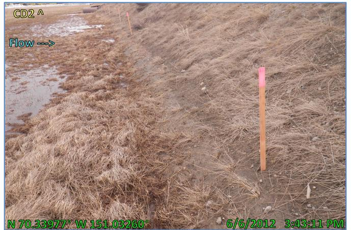
Photo 4.62: Erosion survey CD2 road prism post-breakup, looking west; June 6, 2012
