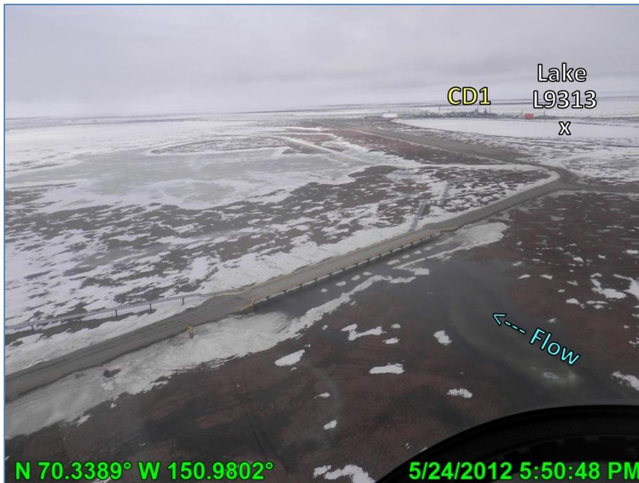
**Photo 2.12: View of south side of long swale bridge with snow mechanically removed prior to breakup and local melt in area, looking east; May 24, 2012**
