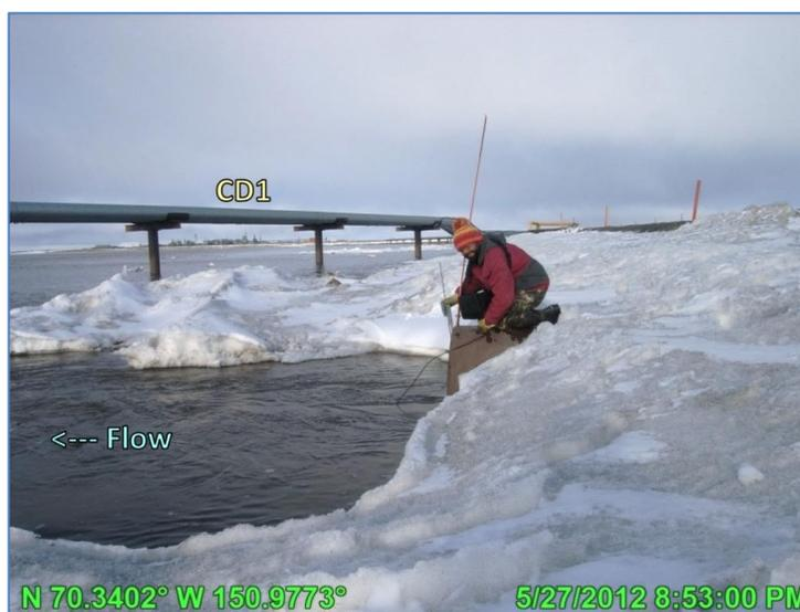
Photo 3.6: Measuring velocity at a culvert along CD2 access road; May 27, 2012
