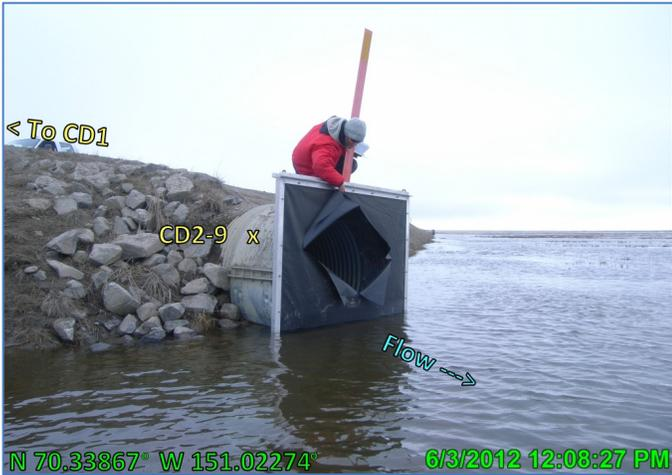
Photo 4.43: CD2 road culvert CD2-9 with fabric cover partially removed, downstream (north) side; June 3, 2012
