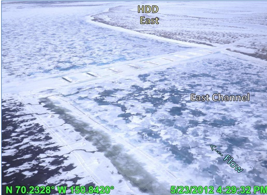
Photo 2.15: Colville River ice bridge crossing slotted to facilitate flood flow prior to breakup, looking downstream (northeast); May 23, 2012
