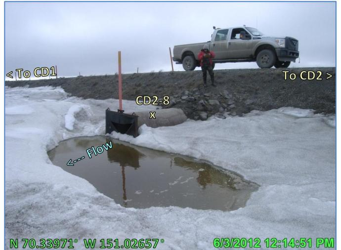
Photo 4.42: Snow removed from outlet area of CD2 road culvert CD2-8 with significant quantities in surrounding vicinity, downstream (north) side; June 3, 2012
