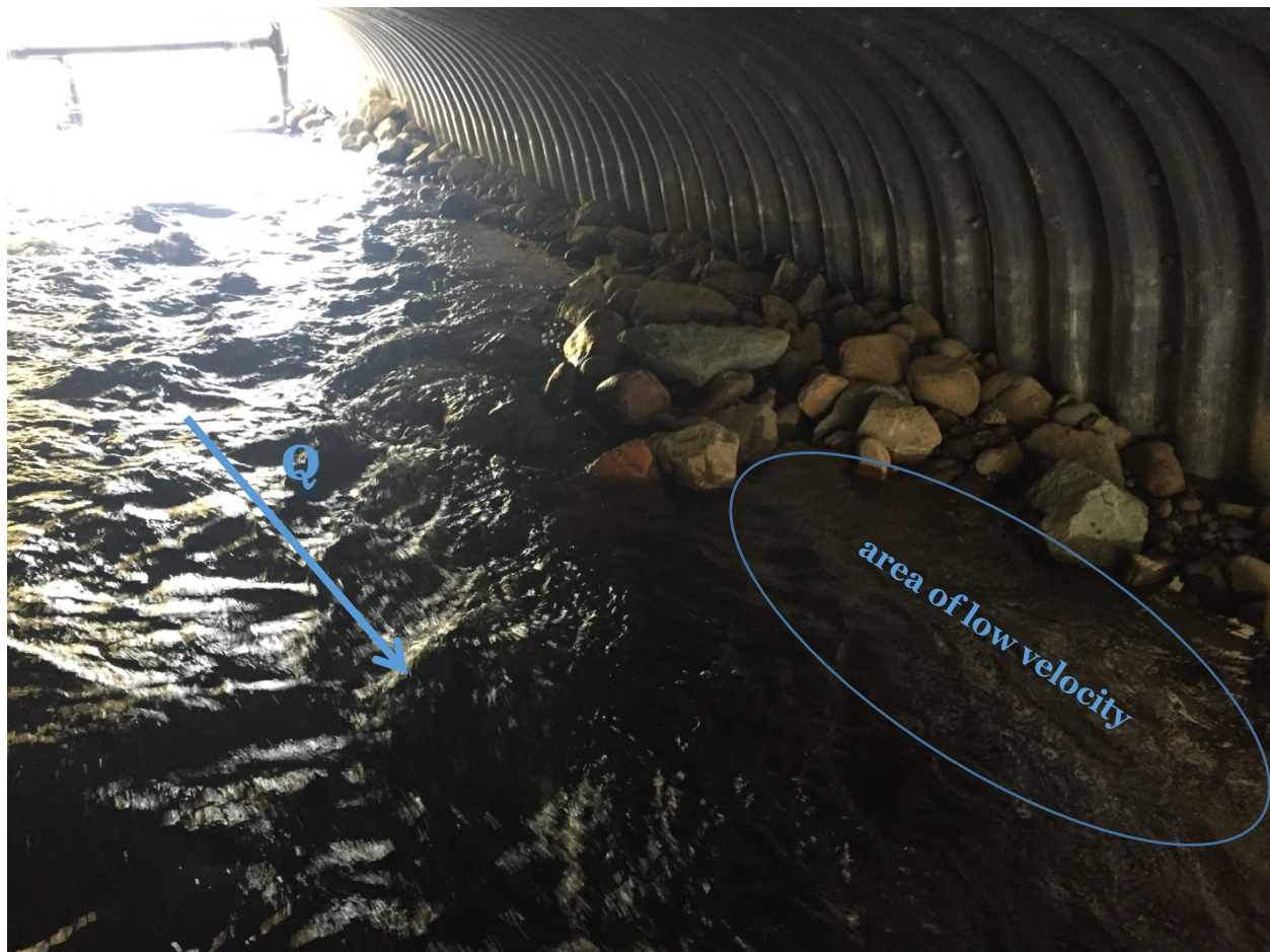
Figure 17. Flow variations inside structure at installed bank
