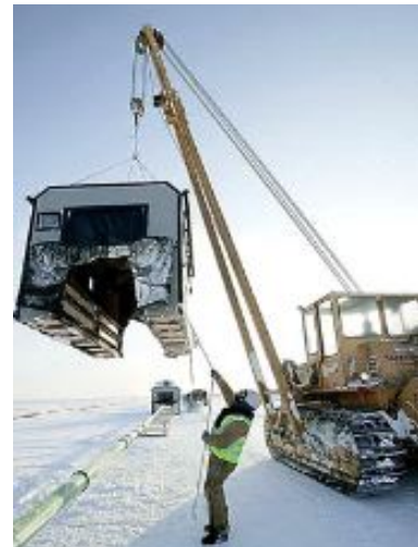
Figure 6: A sideboom tractor lifts a welding shack during pipeline assembly (Bradner 2007).
