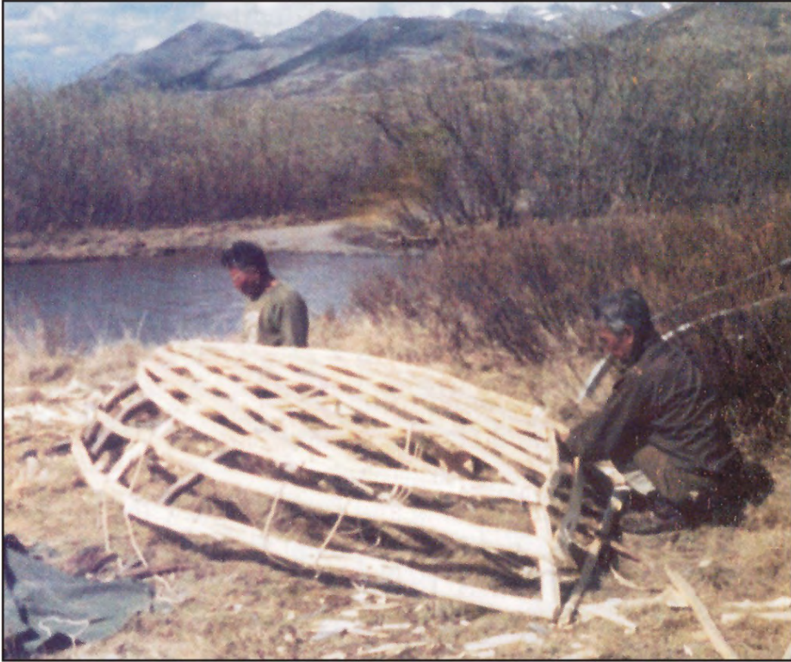
Figure 14. Kwethluk hunters lashing frame members together for a bear skin boat on The Kwethluk River, 1988. Photo by John W. Andrew, reprinted from Alaska Fish and Game , November-December 1989, Vol. 21, No. 6, p. 12.
