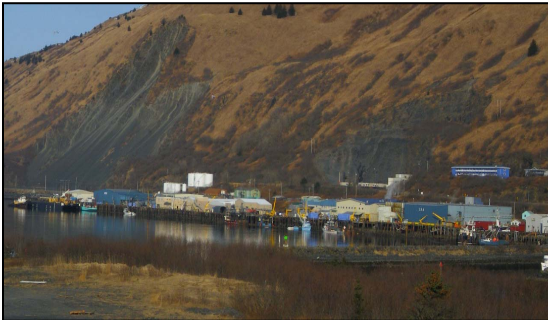
Figure 4-4 Industrial Zone in Kodiak City, 2010
