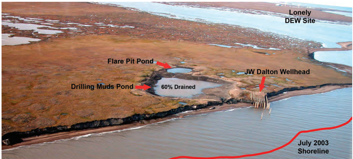
Figure 4-4. JW Dalton well site on the Beaufort Sea coast, National Petroleum Reserve-Alaska (NPR-A). Photograph taken by S. Flora, Bureau of Land Management, September 2004. Approximately 100 m of coastal erosion occurred at this site during the summer of 2004.
